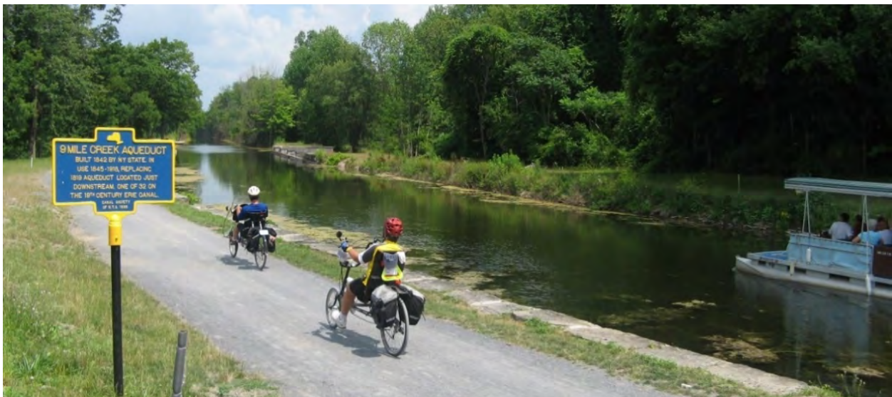
Cyclists on a restored stone and wood aqueduct of the Erie Canal over Nine Mile Creek in Camillus, New York. (Photo: PTNY)
