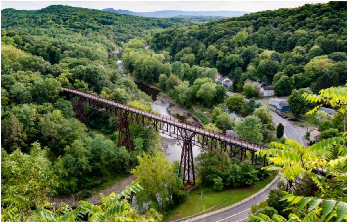
Restored Rosendale Trestle on the Wallkill Valley Rail Trail
