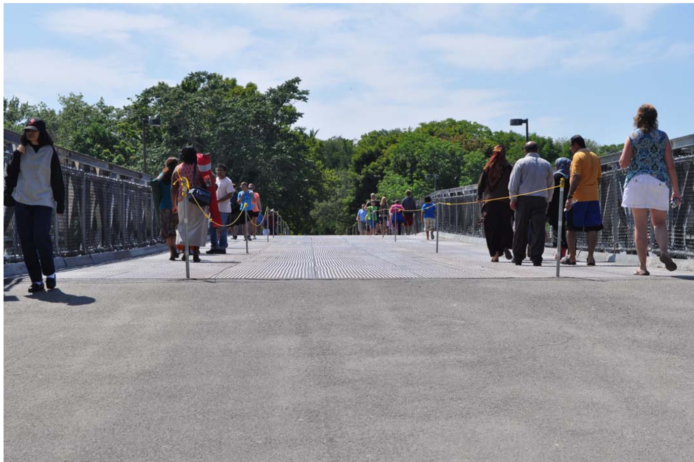
Figure 1.2.1.c Existing Conditions BIN 5522000 (Mainland to Green Island)
