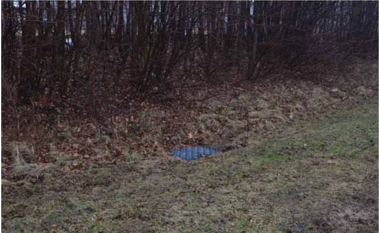
Photograph 8. Storm drain opening in Survey Area 3, facing southeast ( Panamerican 2016 ).
