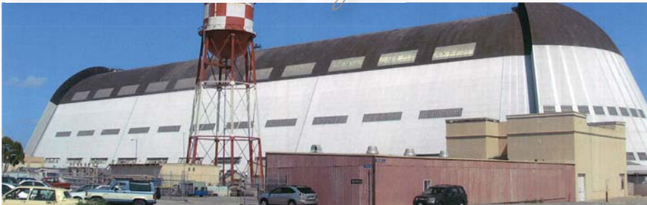
Hangar I, a historic dirigible hangar at Moffett Field at NASA Ames Research Center, California
