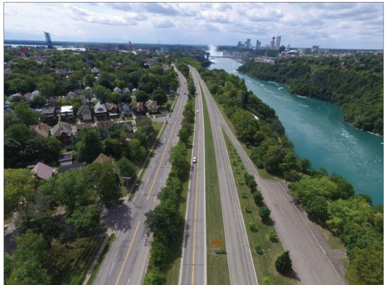
Existing RMP and the Project Study Area Looking South
