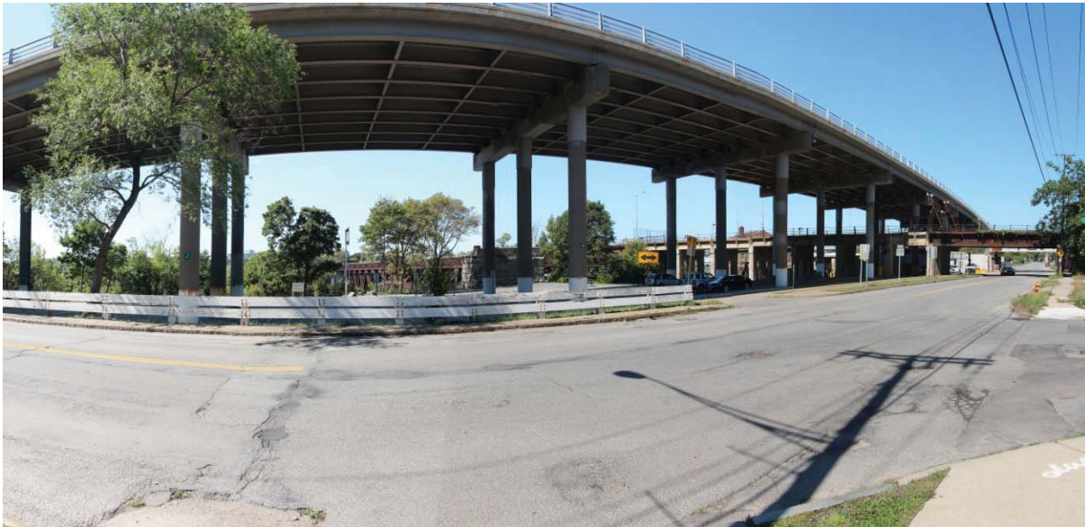
Existing / No-Build Alternative – View toward the RMP Viaduct from intersection of Whirlpool Street and Ontario Avenue
