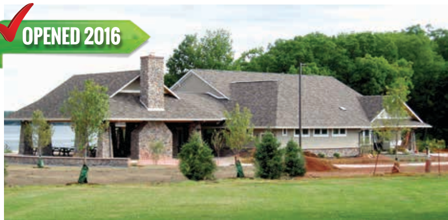
Campers staying at one of the park system’s largest campgrounds now have a quality bathhouse at Wellesley Island State Park (below).
