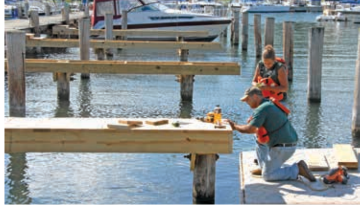
Workers repair docks at Seneca Lake State Park.
