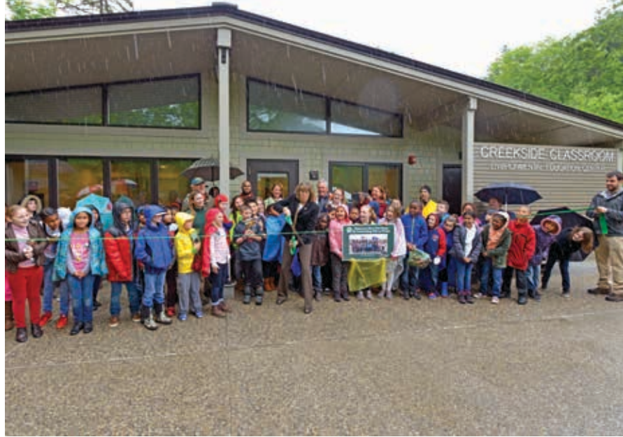
The Creekside Classroom project transformed an old comfort station into classroom space for the park's environmental education program.
