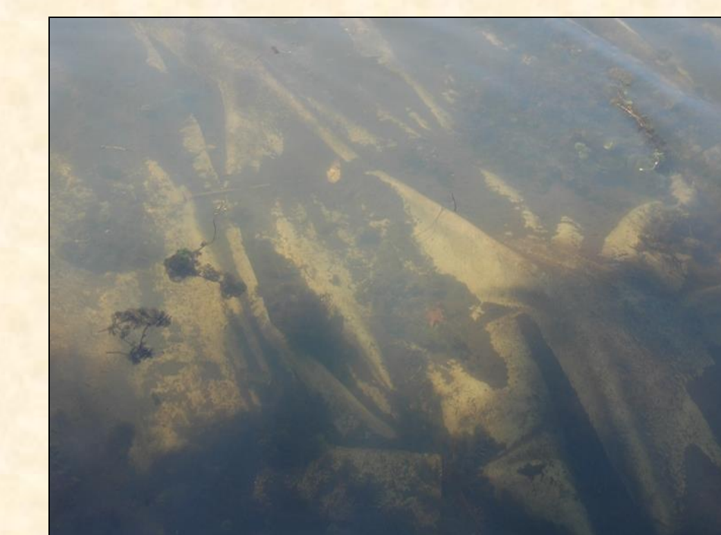
Sediment Buildup On Barrier
