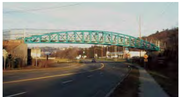
Gateway Bridge over N. Y. S. Rtes 13/34/96
