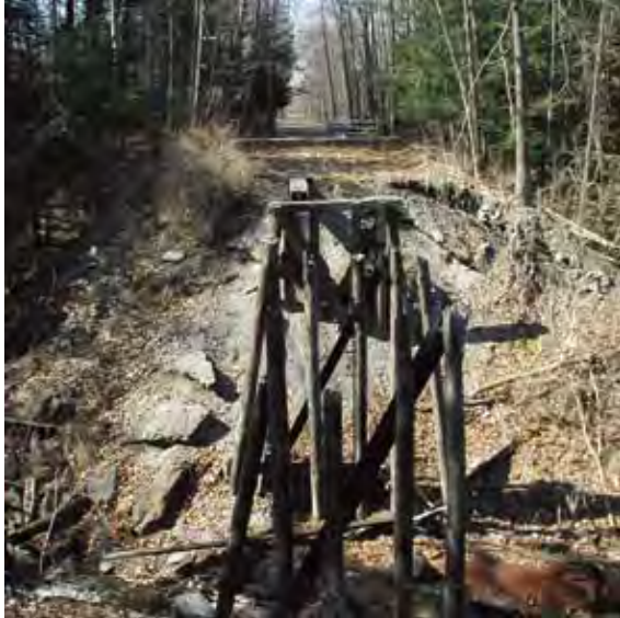
Remains of railroad trestle crossing Glenwood Creek
