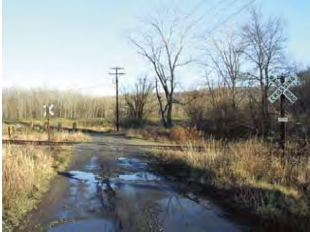
Existing at-grade crossing of the active low-traffic Norfolk Southern Line
