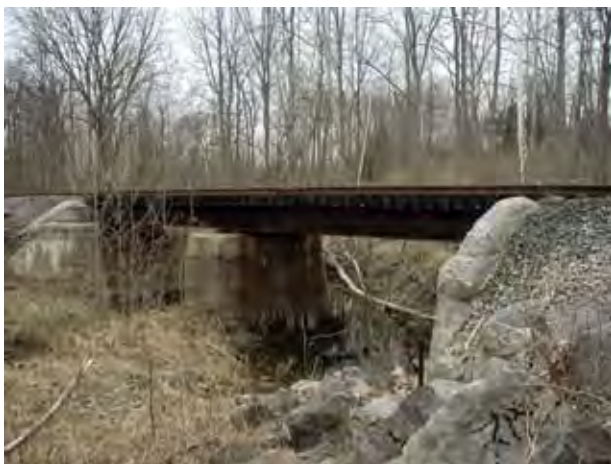
Rail bridge that can accommodate a trail underpass
