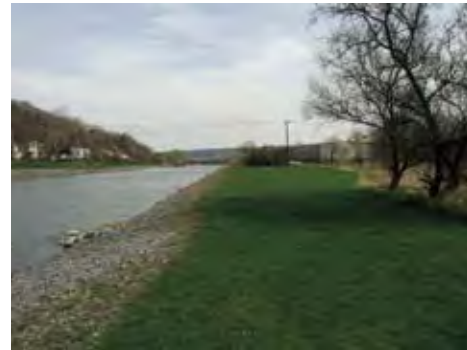
Cayuga Inlet Flood Control Channel
