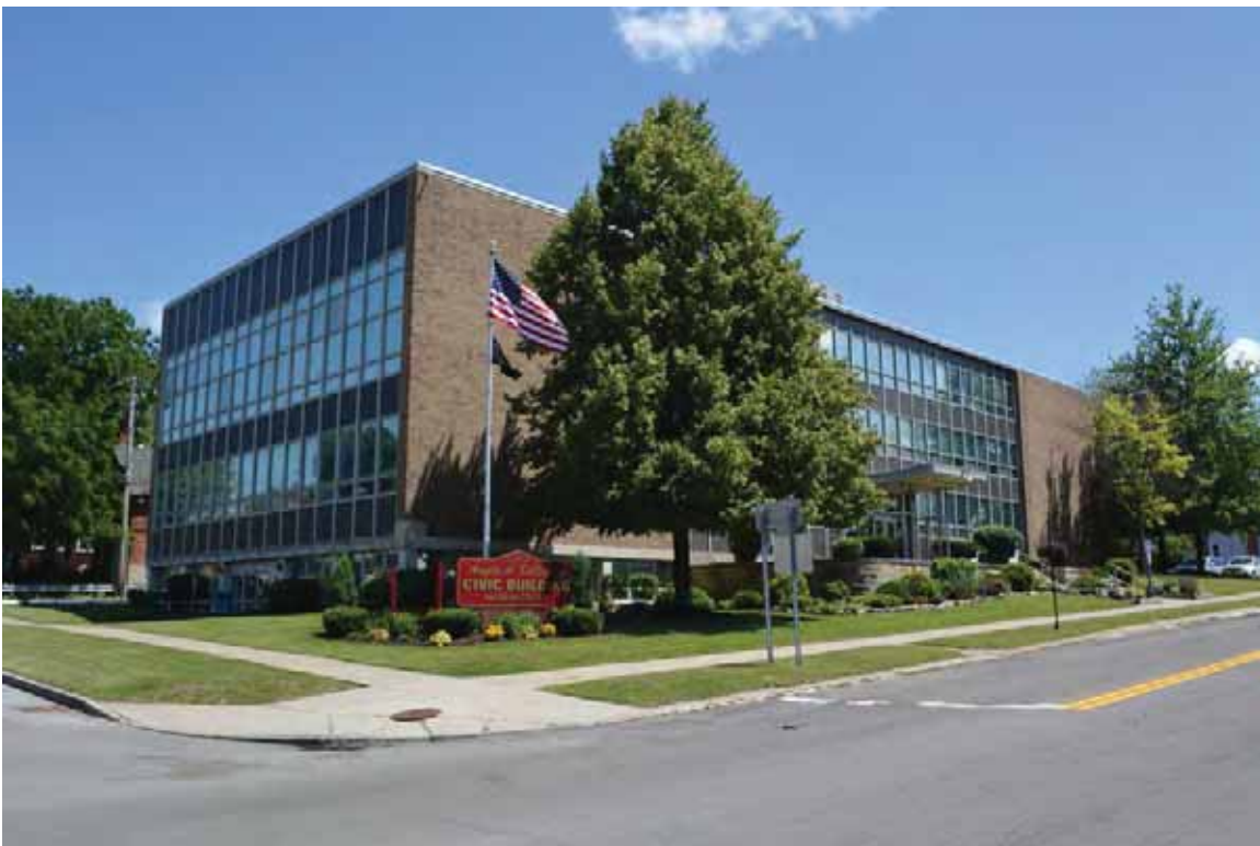
Photograph 1. Niagara County Building, facing southeast ( Panamerican 2014 ).
