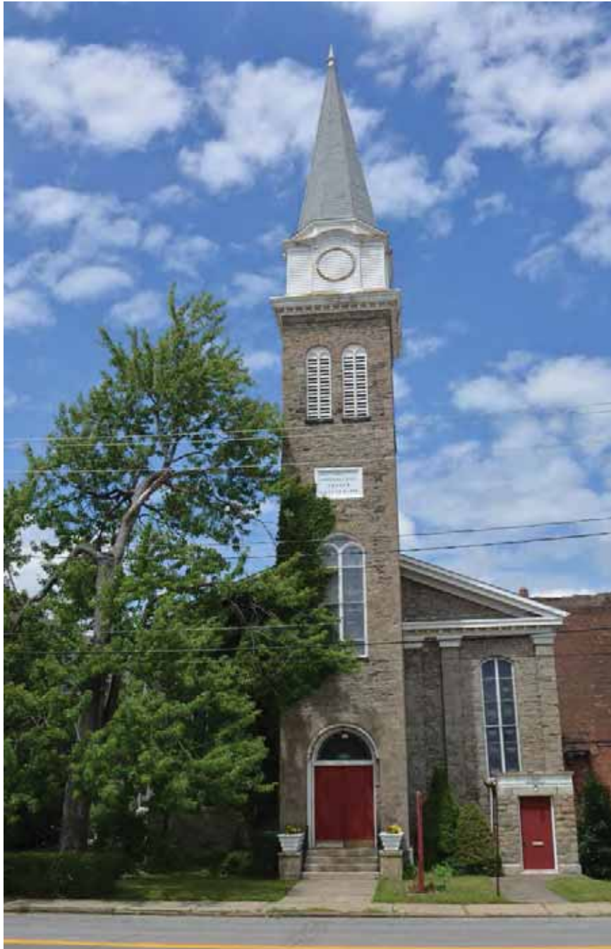
Photograph 1. First Congregational Church at 822 Cleveland Ave (left), facing north ( Panamerican 2014 ).
