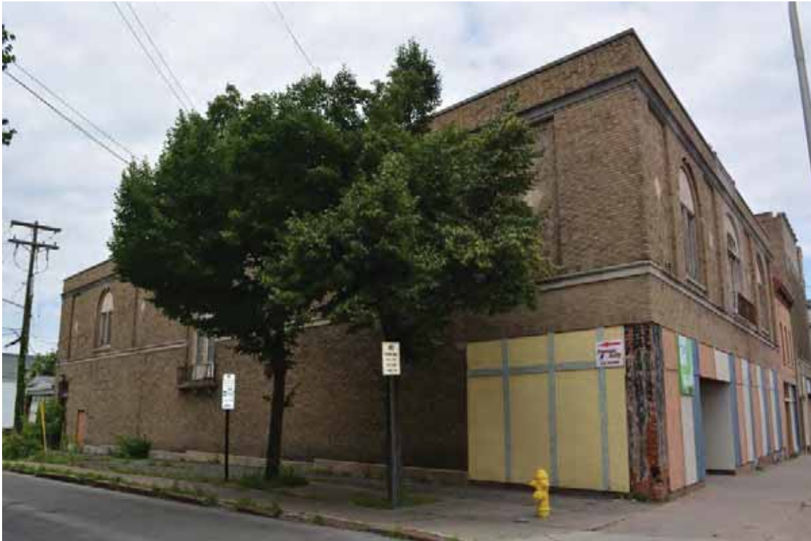
Photograph 2. 1802 Main Street, facing northwest ( Panamerican 2014 ).
