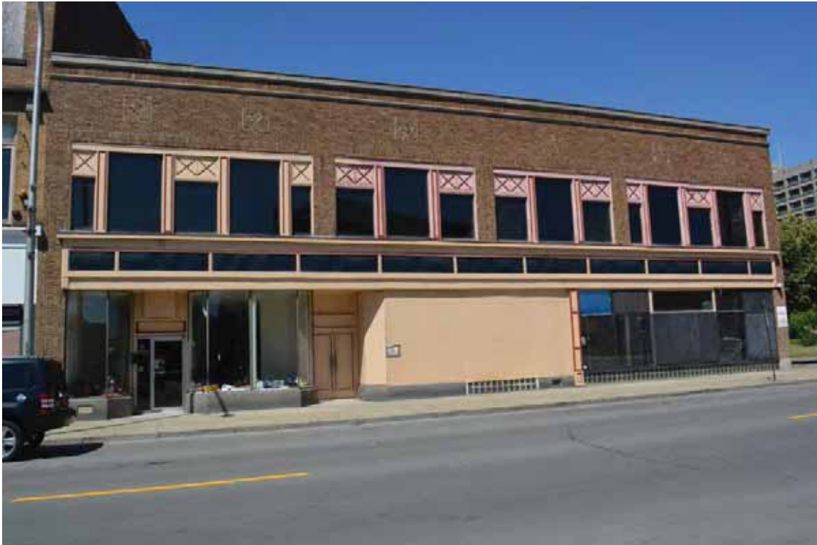
Photograph 2. 855 Niagara Ave, facing west ( Panamerican 2014 ).
