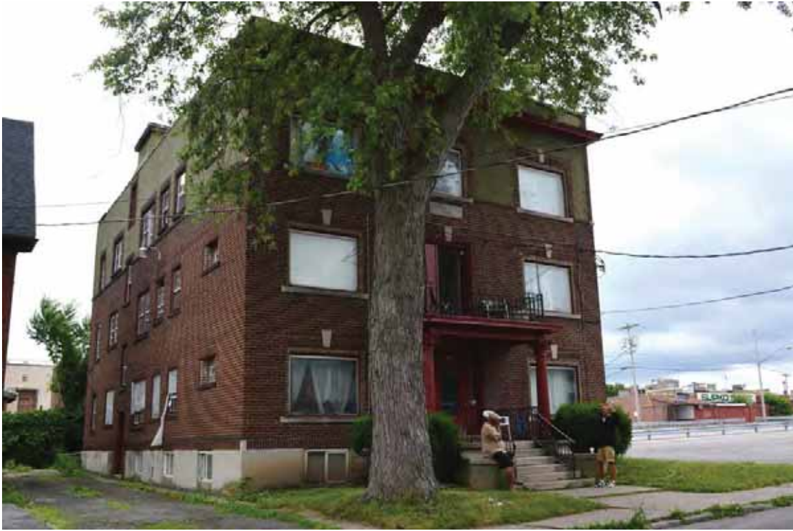
Photograph 2. LaRose Apartments at 1643 Eight St, facing southeast ( Panamerican 2014).
