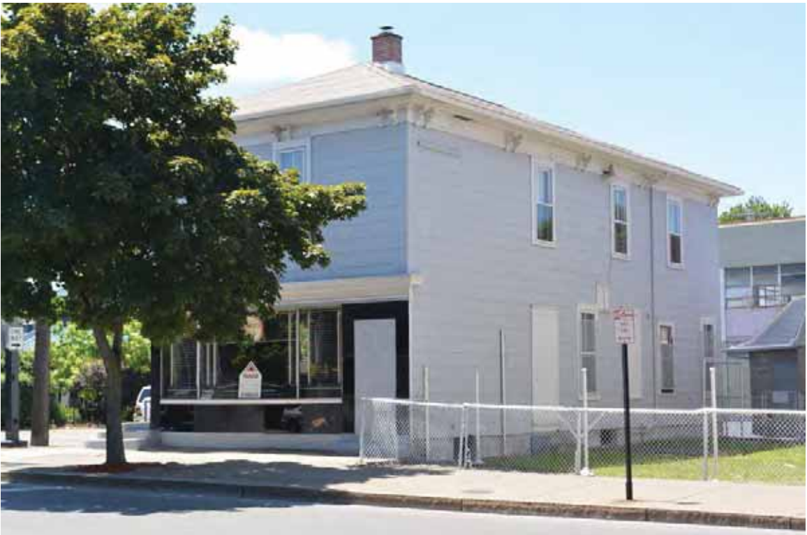
Photograph 2. 1402 Main St, facing southwest ( Panamerican 2014 ).
