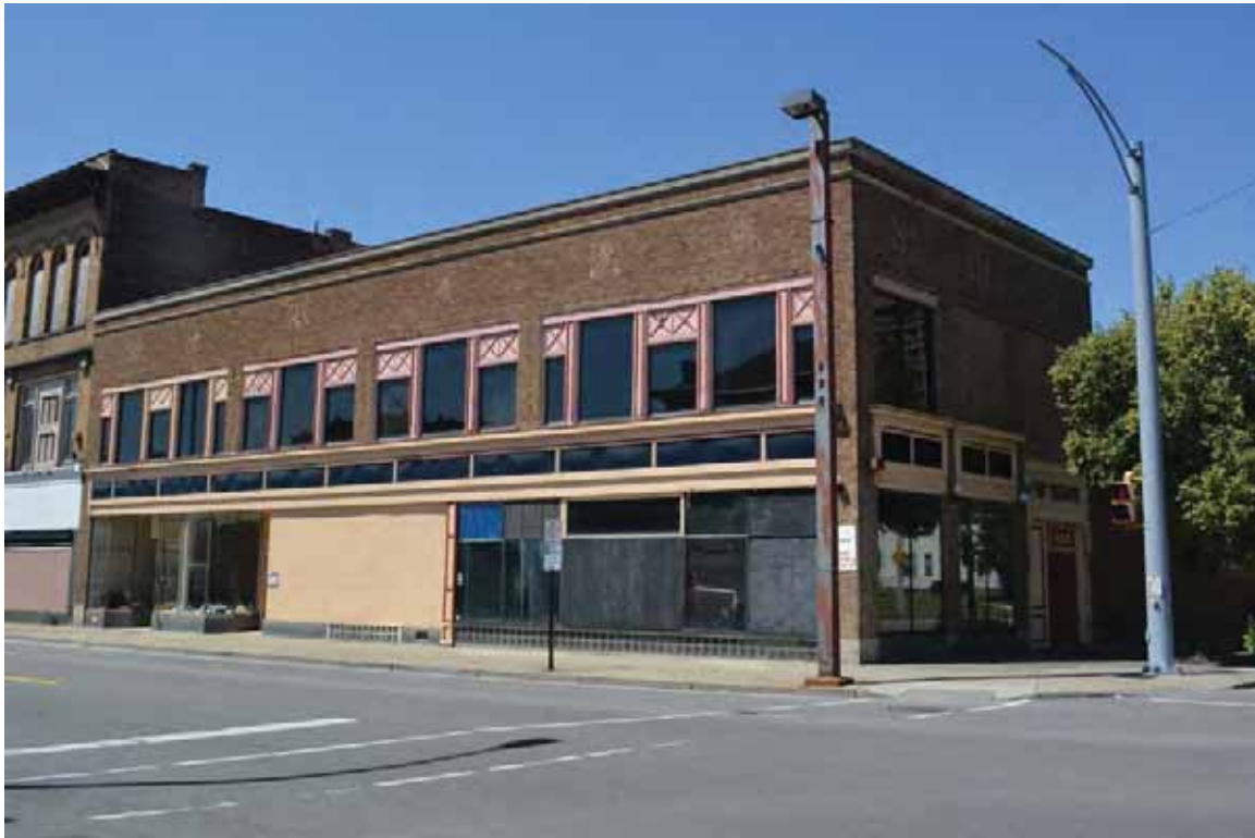
Photograph 1. 855 Niagara Ave, facing southwest ( Panamerican 2014 ).
