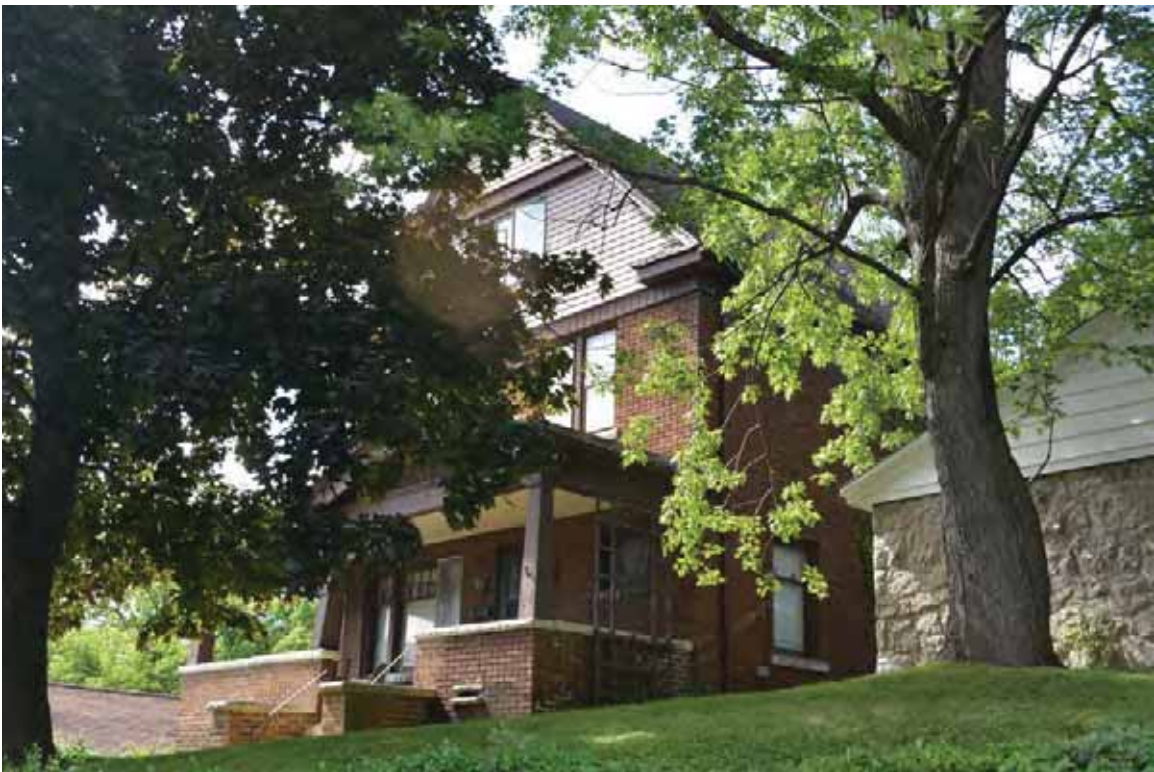
Photograph 3. Residence at 616 Chasm Ave, facing north west (PCI 2014) .
