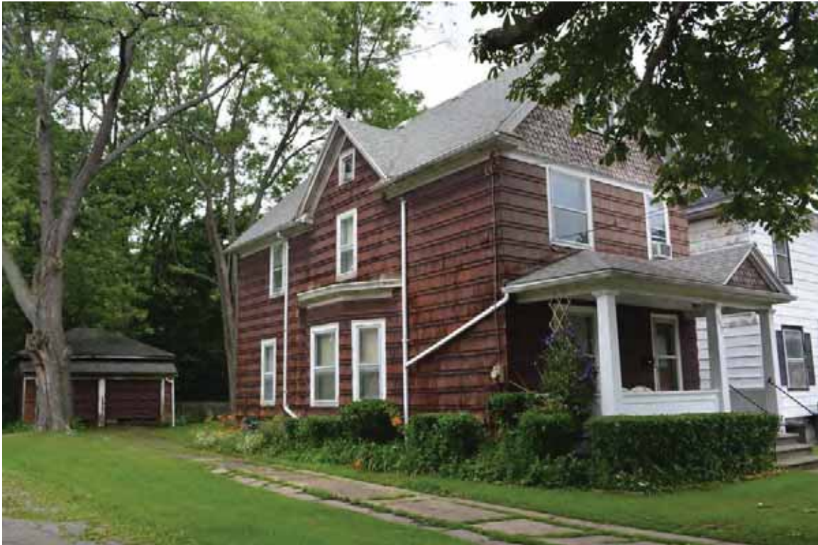
Photograph 2. 1412 Eighth Street, facing northwest southeast ( Panamerican 2014 ).
