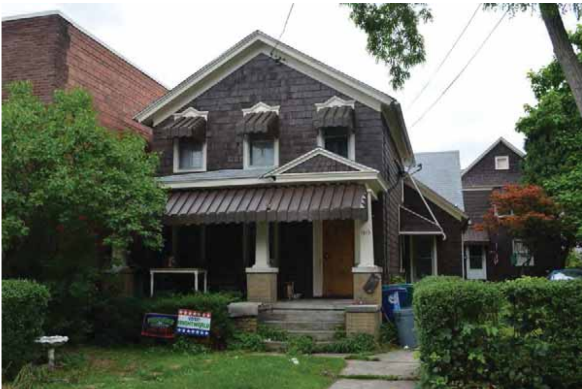
Photograph 1. Residence at 1511 Eighth Street, facing northeast ( Panamerican 2014 ).
