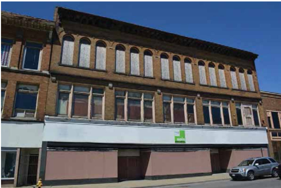
Photograph 1. 2018 Main St, facing west-northwest ( Panamerican 2014 ).
