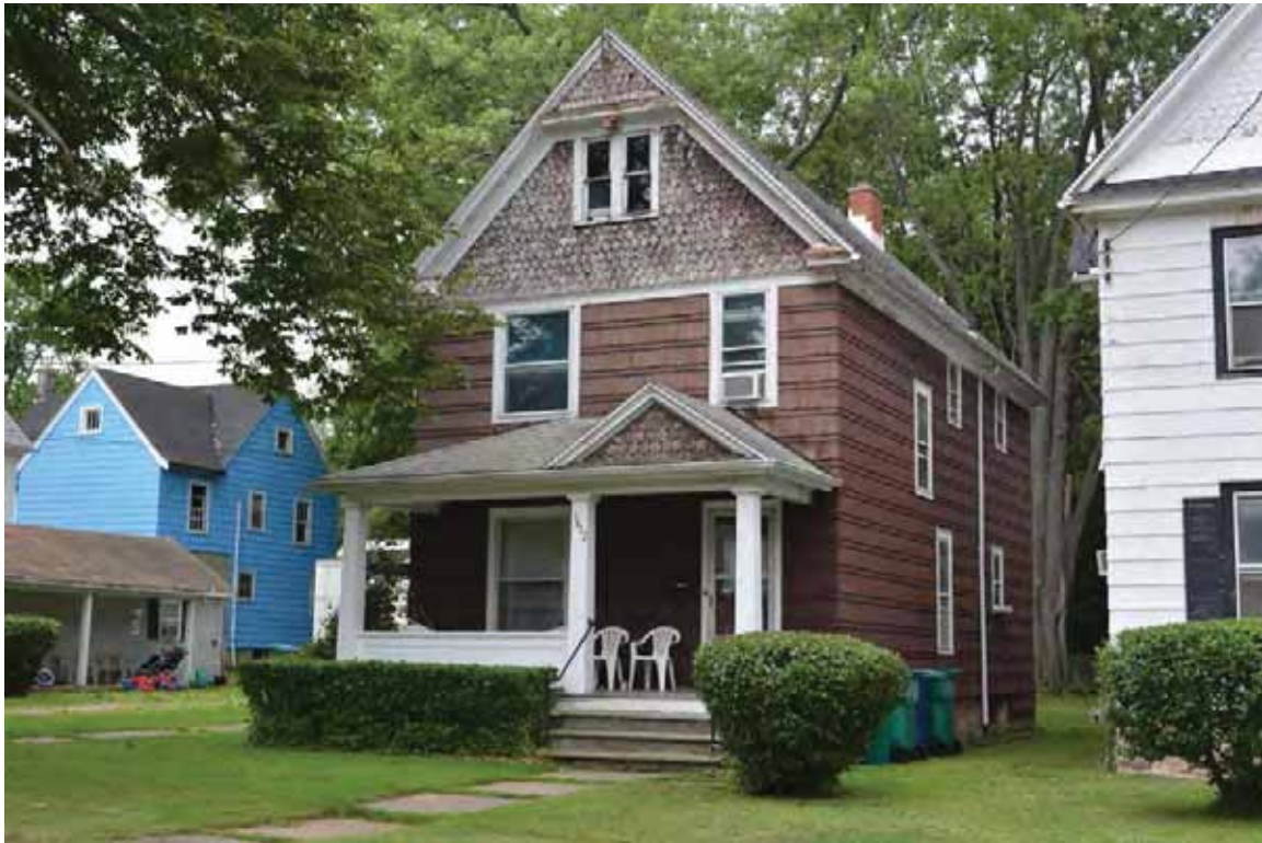
Photograph 1. 1412 Eighth Street, facing southwest ( Panamerican 2014 ).
