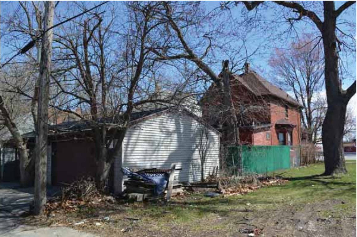
Photograph 3. Residence at 1618 Eighth Street, facing northeast ( Panamerican 2015 ).
