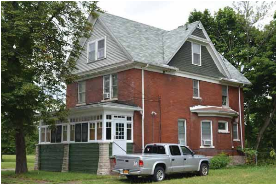
Photograph 1. 734 Willow Ave, facing northwest ( Panamerican 2014 ).
