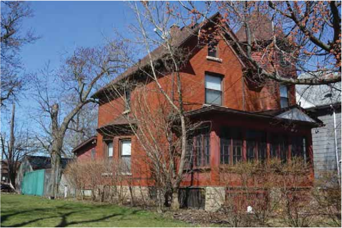
Photograph 2. Residence at 1618 Eighth Street, facing northwest ( Panamerican 2015 ).
