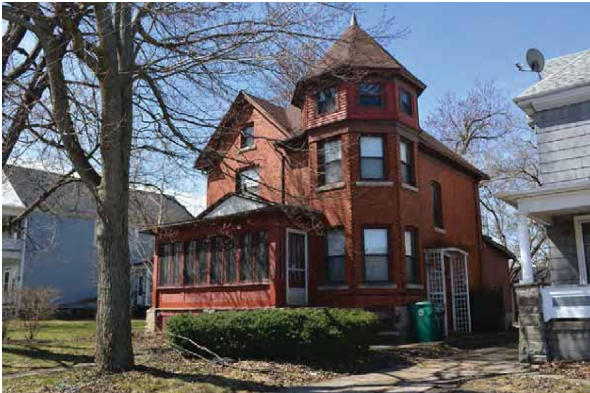
Photograph 1. Residence at 1618 Eighth Street, facing southwest ( Panamerican 2015 ).
