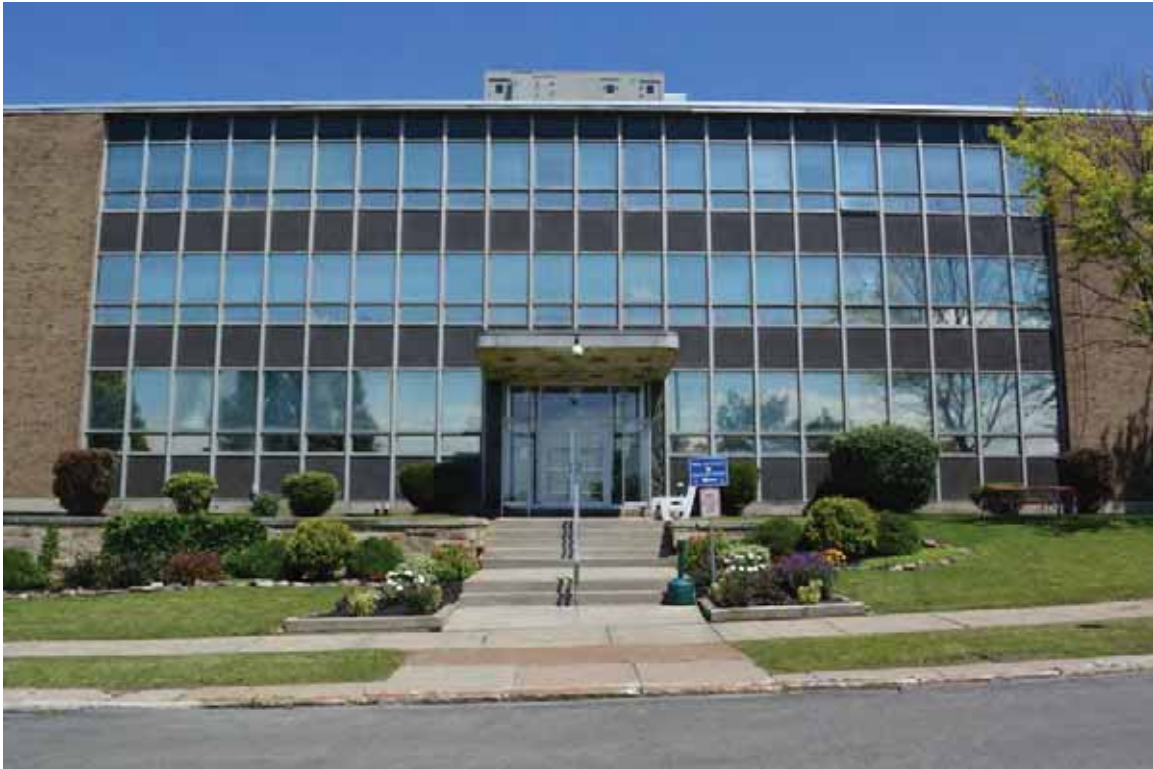
Photograph 2. Niagara County Building, facing east ( Panamerican 2014).
