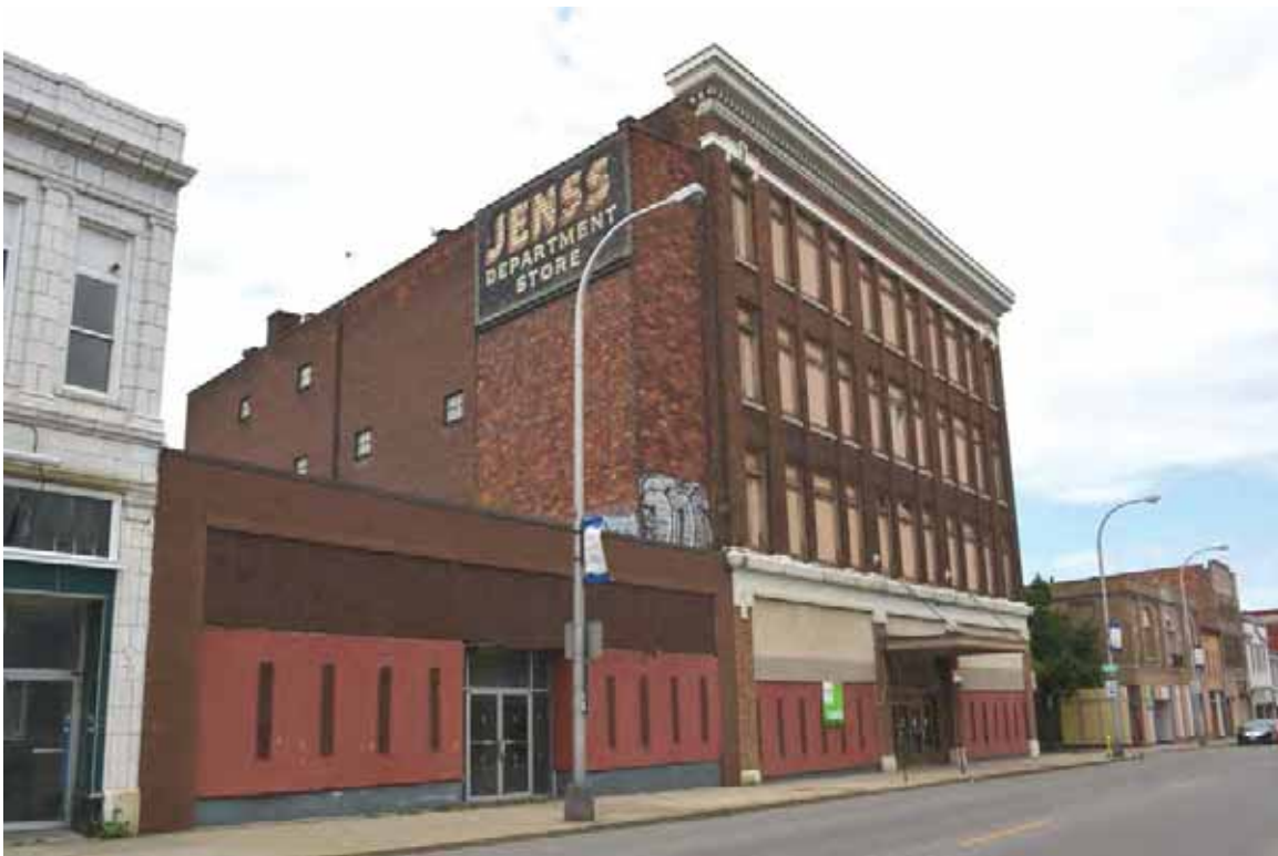
Photograph 2. 1708 Main St., facing northwest ( Panamerican 2014 ).
