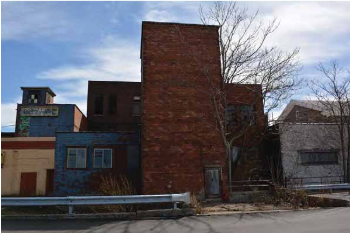
Photograph 2. 2018 Main St, facing east ( Panamerican 2014 ).
