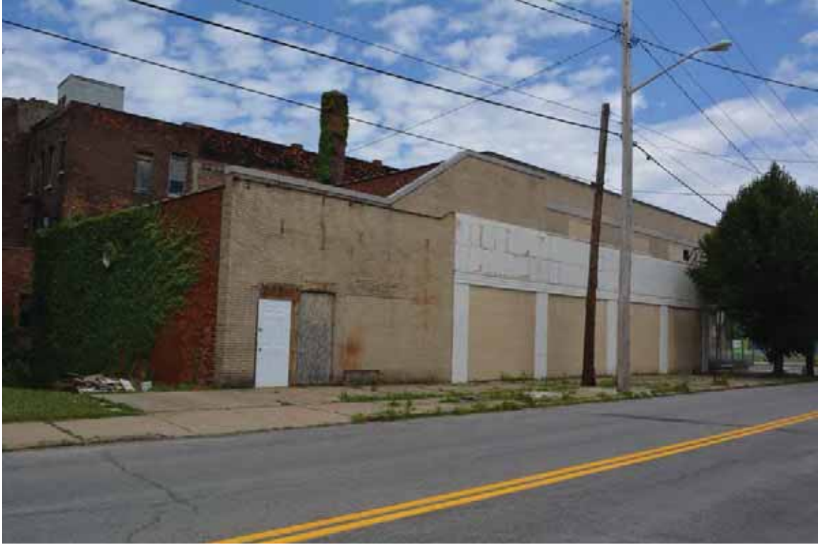
Photograph 6. 2002 Main St, facing northeast ( Panamerican 2014 ).
