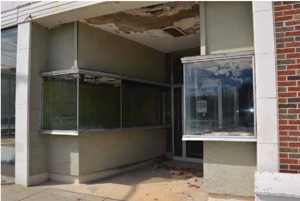
Photograph 5. 2002 Main St, facing southwest ( Panamerican 2014 ).
