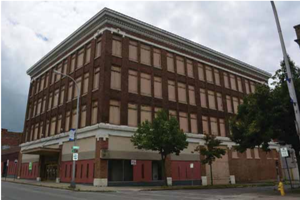
Photograph 1. 1708 Main St., facing southwest ( Panamerican 2014 ).
