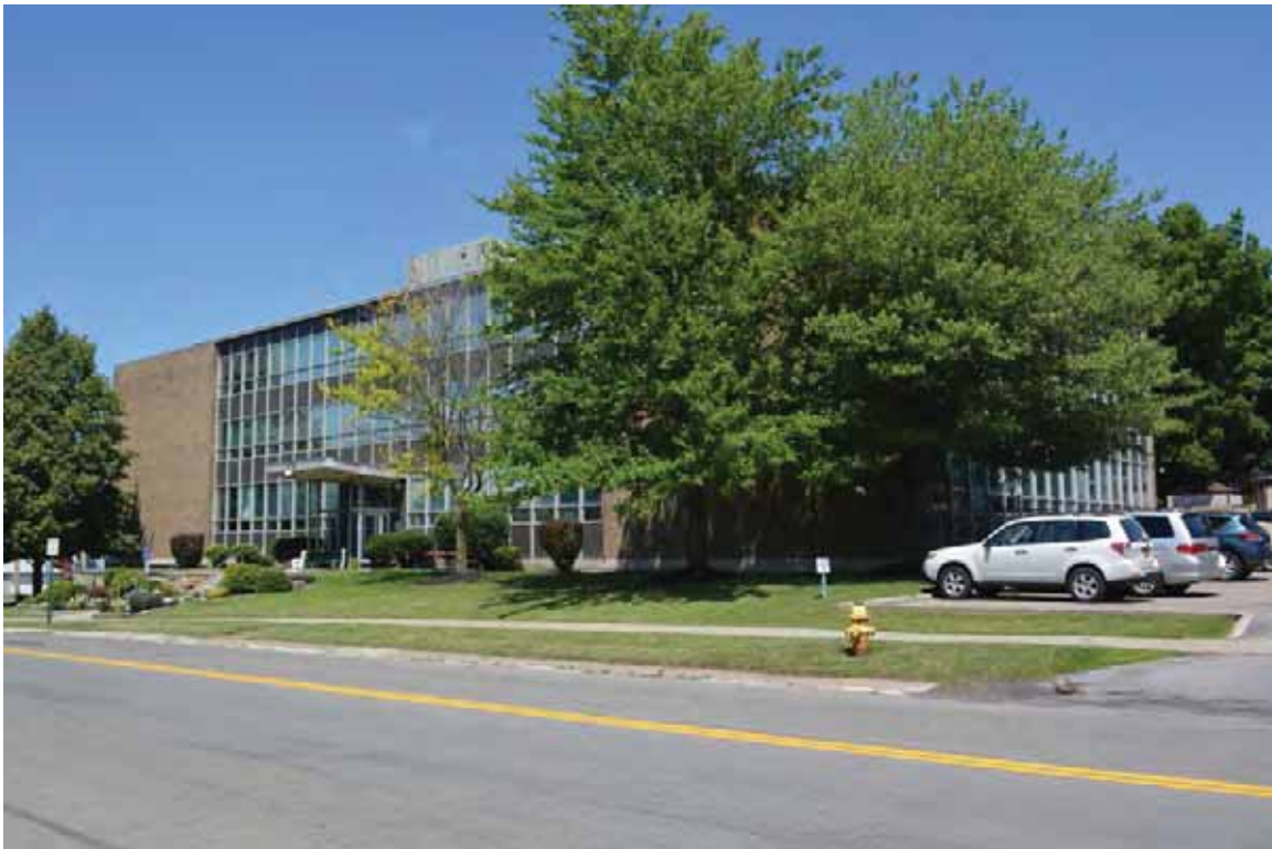
Photograph 3. Niagara County Building, facing northeast ( Panamerican 2014).
