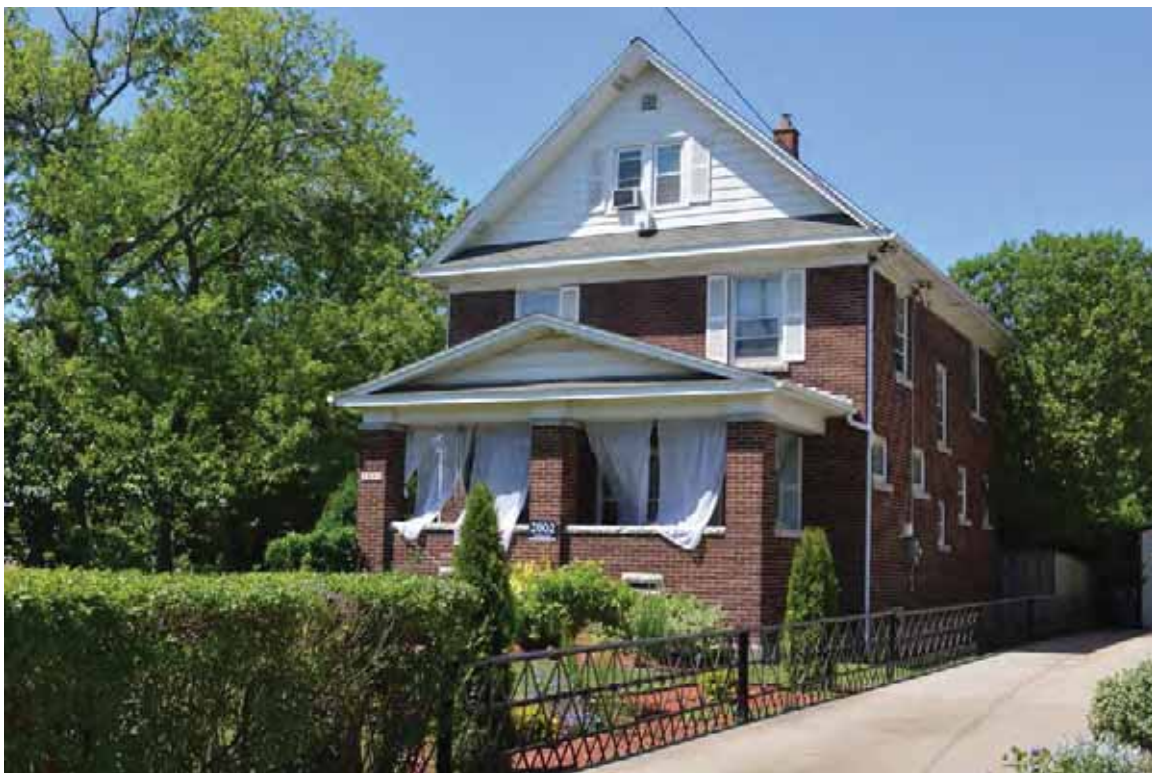
Photograph 1. Residence at 2802 Lewiston Road, facing west-southwest ( Panamerican 2014 ).
