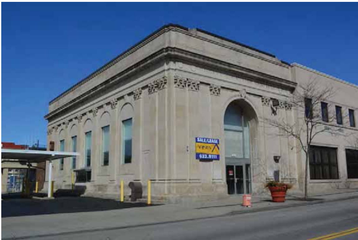
Photograph 1. Old Niagara County Savings Bank, facing northwest ( Panamerican 2015 ).
