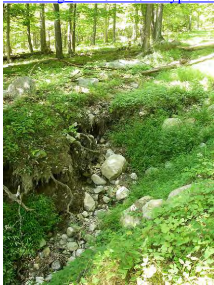
Awosting_PN4 9-4-09 waypoint 16 serious erosion
