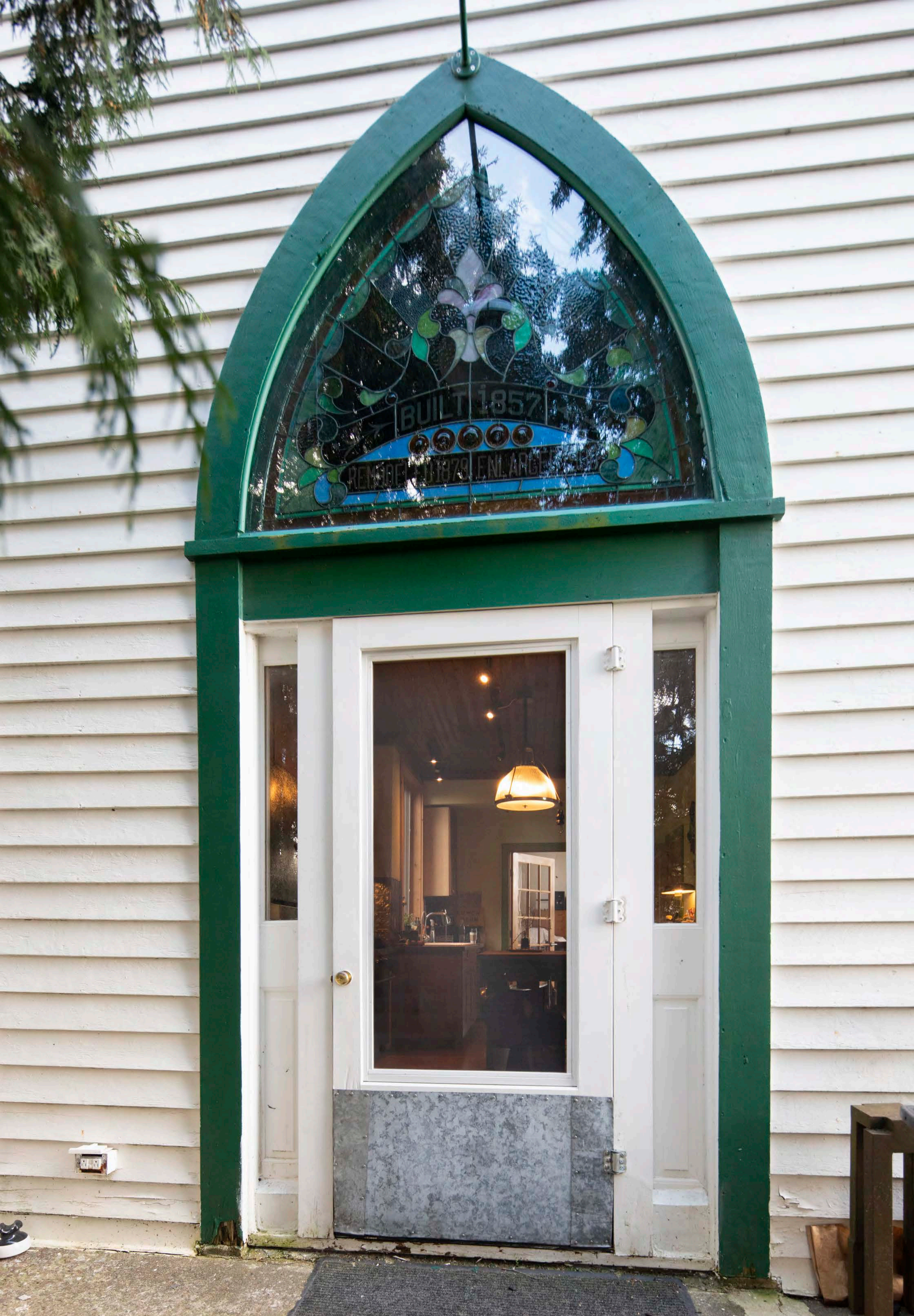
ME Church, main entry door, with stained glass window, to south.
