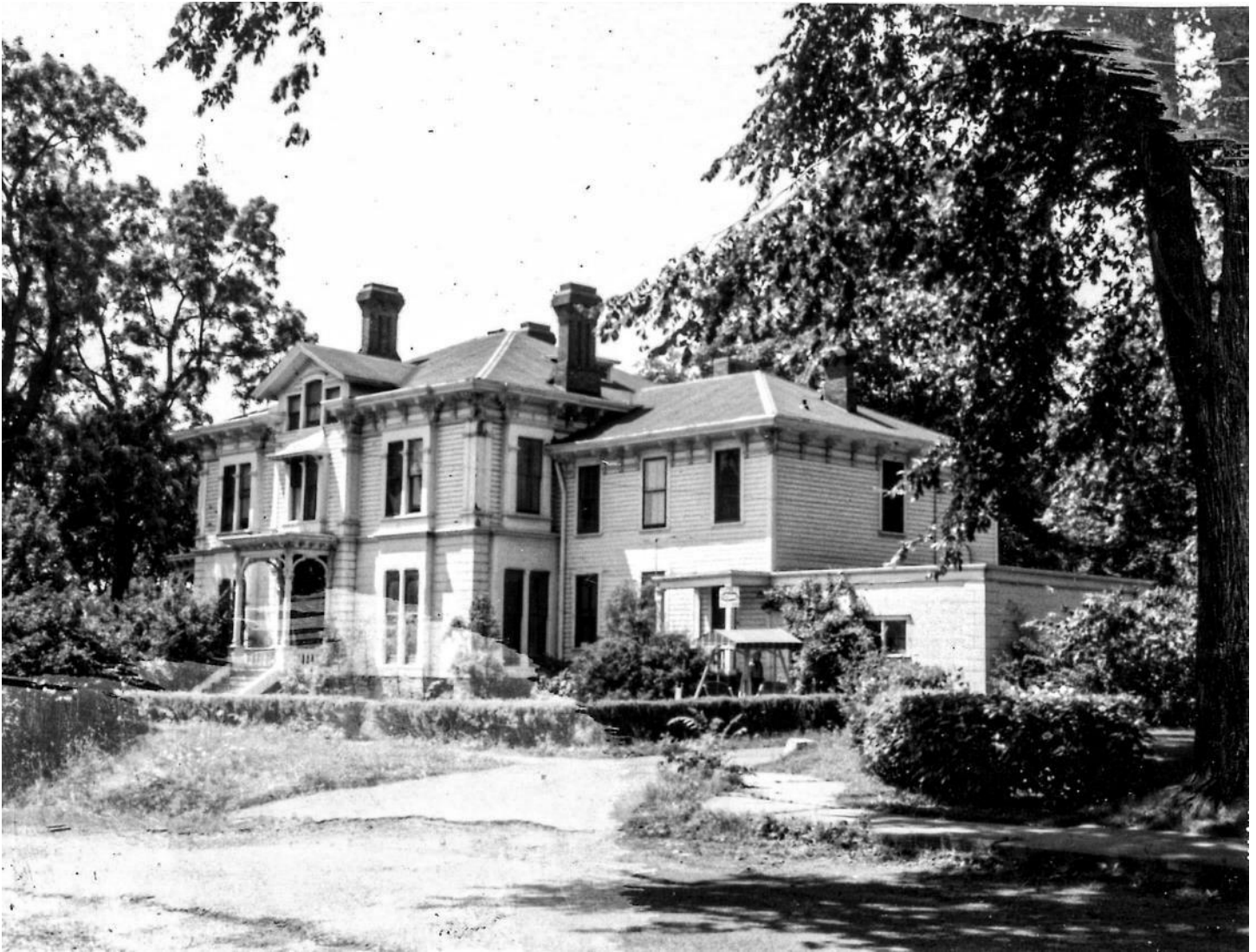
Figure 6. Undated photograph of the Tatler Club prior to the installation of aluminum siding in 1963 (Tatler Club private collection). Facing Southwest.
