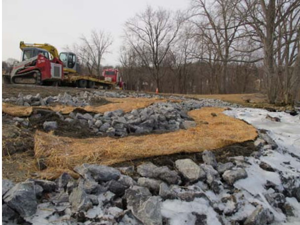
Figure 2: The site following construction in February 2012.
