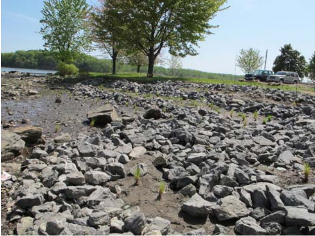
Figure 3: The site immediately after planting, note the small plants between rock terraces.
