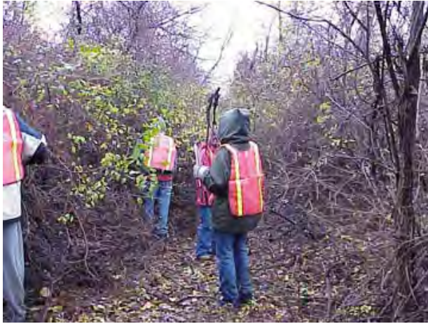
In October 2000, volunteers helped with the initial clearing of a segment of the trail corridor near Taughannock Falls State Park to prepare it for future development.
