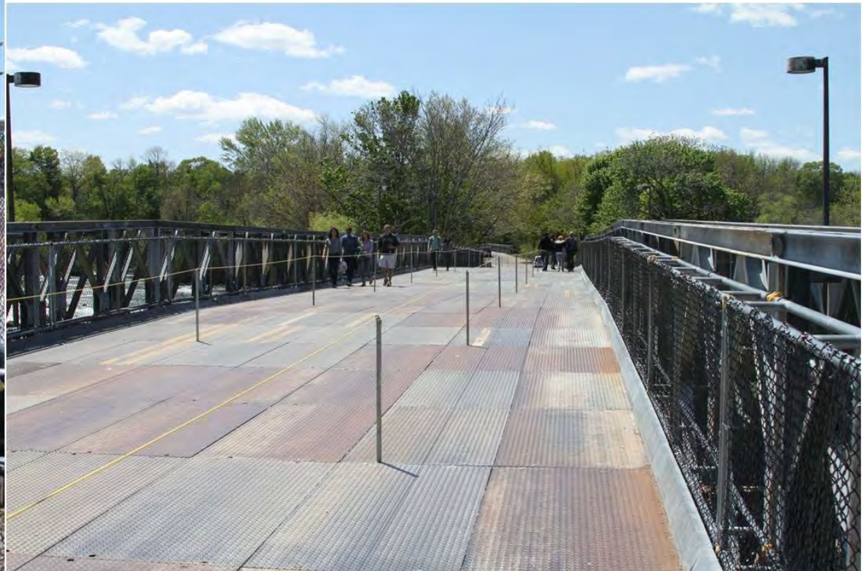
Temporary Mabey Truss Bridge
