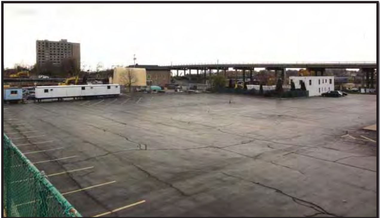
Photograph 1.18. View of the Whirlpool Rapids Bridge, Robert Moses Parkway overpass, restored Custom House and site of the new train station, presently under construction, from Lewiston Road/Main Street, facing southwest (Panamerican 2014).
