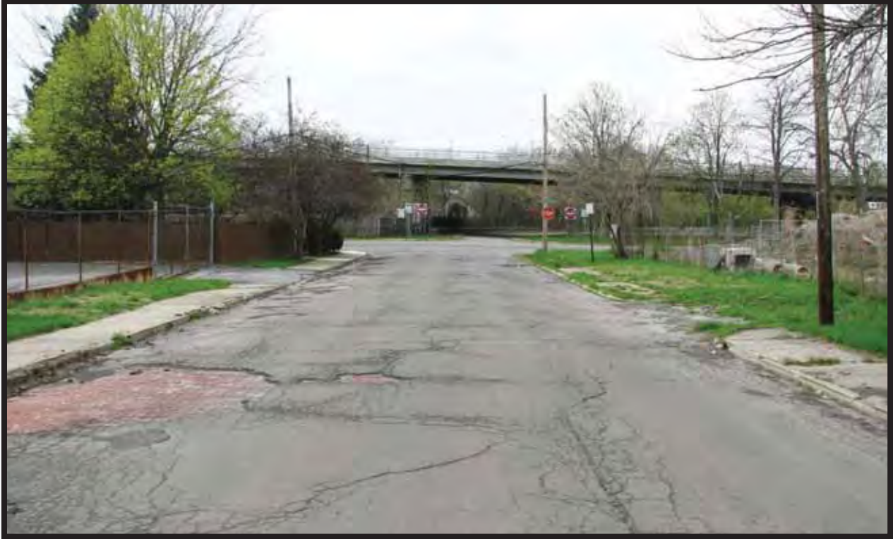
Photograph 1.43. View of Bellevue Avenue toward Whirlpool Street, facing west-southwest ( Panamerican 2015 ).
