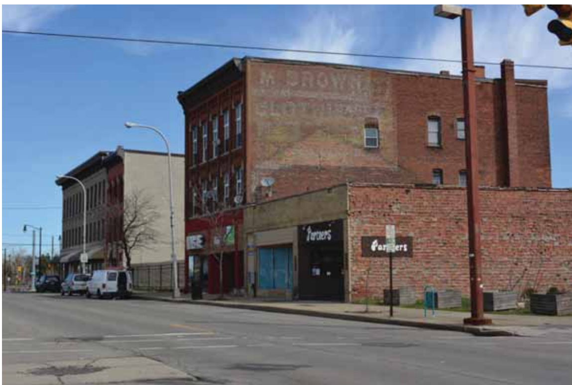
Photograph 4.7. North end of the proposed Upper Main Street Historic District (2107-217 Main Street [outside of study area]) from Niagara Avenue, facing northeast (Panamerican 2015).
