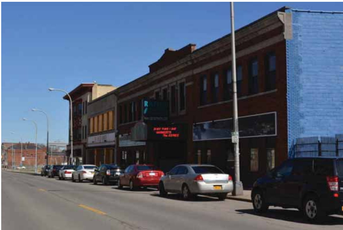
Photograph 4.2. Buildings outside of study area at 1711-1809 Main Street, proposed Upper Main Street Historic District, facing northeast (Panamerican 2015).
