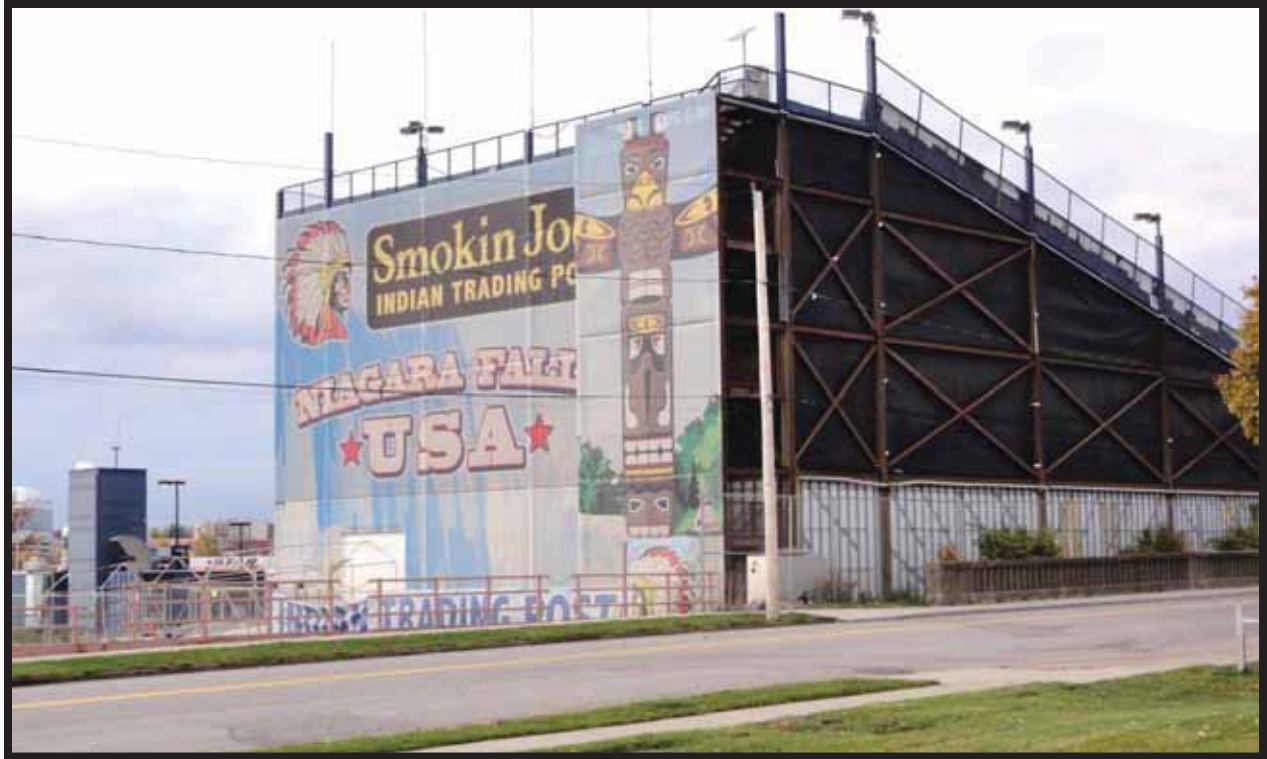
Photograph 1.55. View of across Second Street from Niagara Street, facing northwest (Panamerican 2015).
