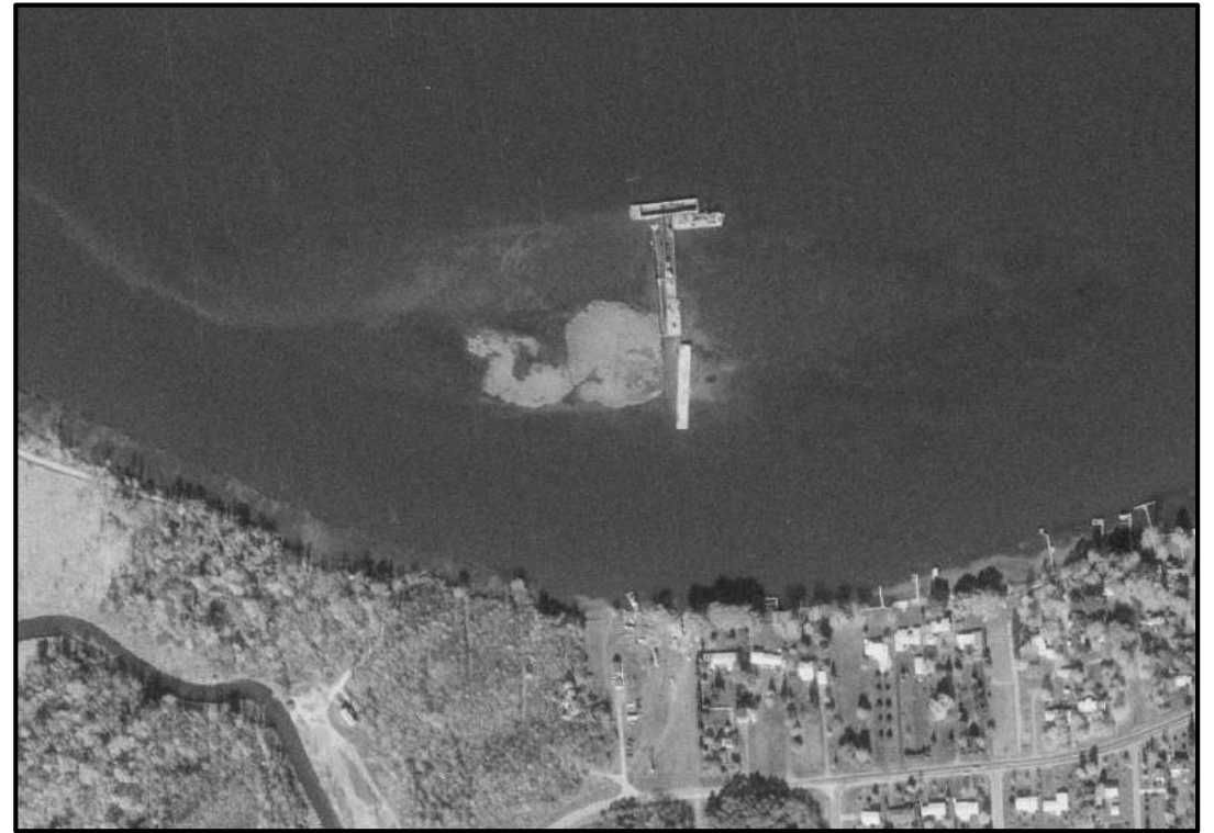
1978-Town of Grand Island Outfall Construction
