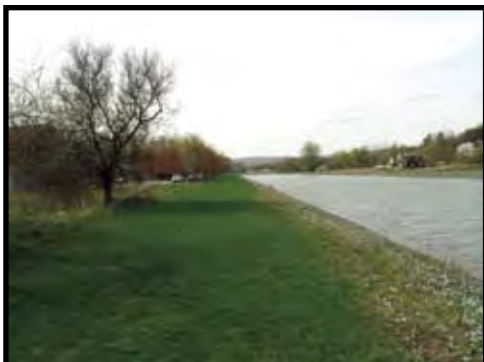
Top of bank along the Cayuga Inlet Flood Control Channel through the City of Ithaca between Buttermilk Falls and Allan H. Treman State Parks/ Cass Park.
