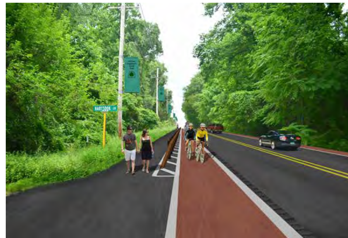
Route 9D at Hartsook Lane, proposed widened roadway with adjacent trail separated by a bikeable shoulder
