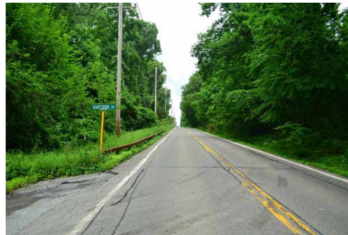
Route 9D at Hartsook Lane, existing condition. View looking north
