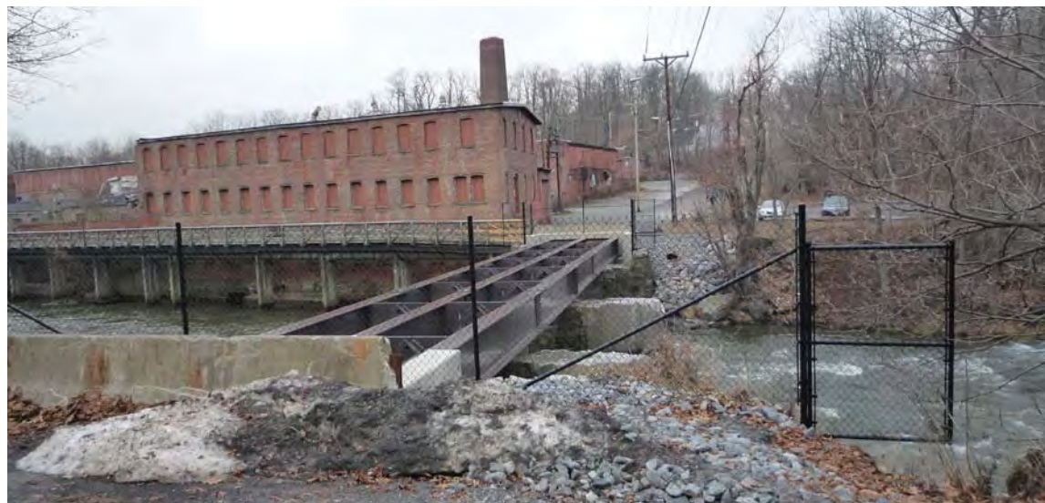
Tioronda Bridge looking north
