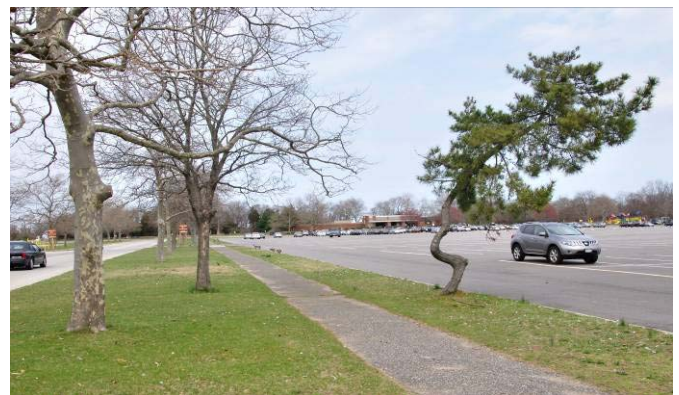
From top to bottom: Cracks in pavement and pooling water; Narrow pathway for pedestrians over bridge; Jogger on Naples Avenue; Trail adjacent to Field 1
