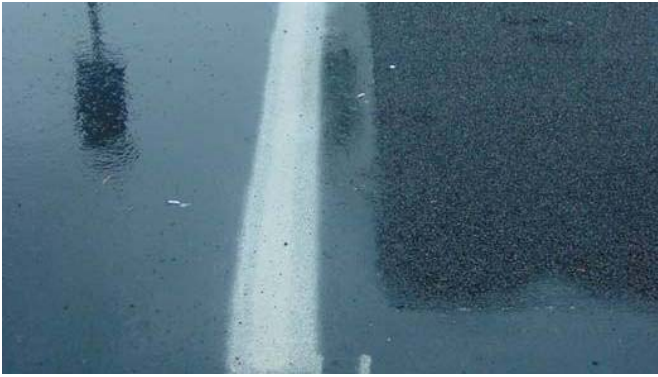
Comparison of traditional asphalt (left) and porous asphalt (on right) (Bassuk, Haffner, and Trowbridge, 2007).
