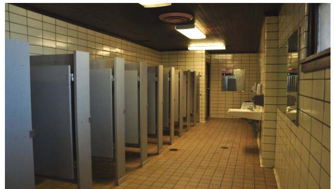
From top to bottom: Field 5 parking lot; Golf course parking lot and clubhouse; Field 4 women's restroom; Field 3 women's restroom
