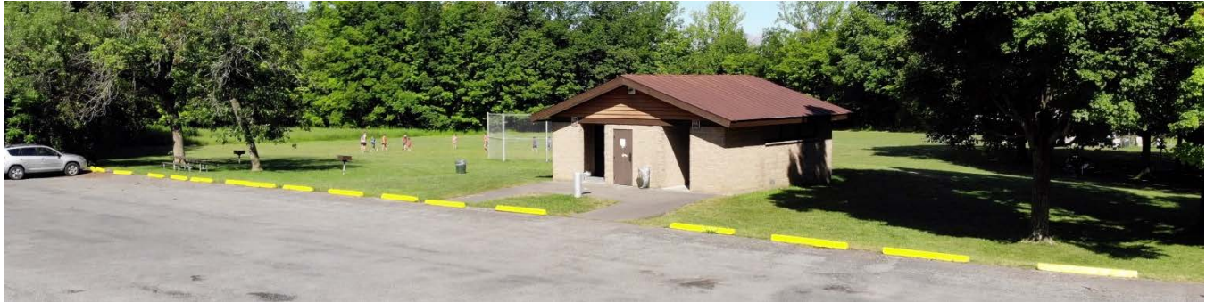
Lakeview Parking Lot
