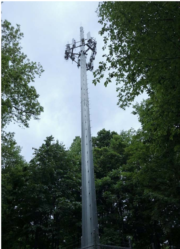
Cellular Tower on the Northern Parcel
