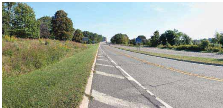
Figure 20: South view of RMP opposite Chasm Avenue
