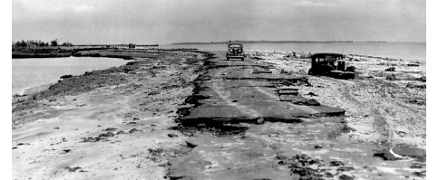
The road into Orient State Park after the storm.
