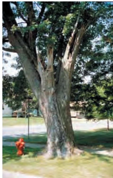
Figure 2.8. This tree has extensive crown dieback, with decayed and broken major limbs. It is a high-risk tree that should be removed.
