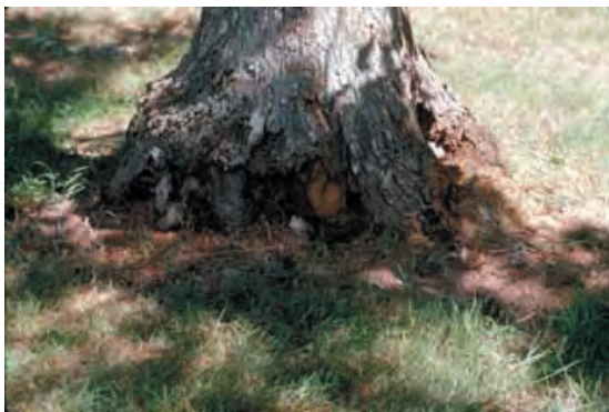
Figure 3.18. Lawn mower damage associated with decay.
