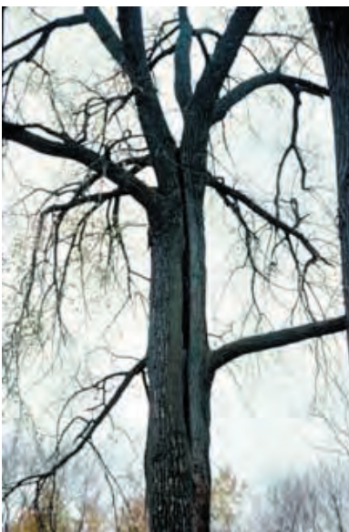
Figure 3.6. Defects are visible signs that a tree has the potential to fail.
