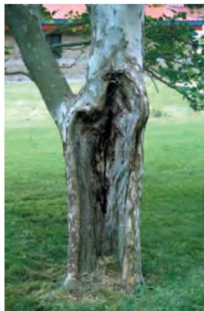
Figure 2.11. The same tree, viewed from the opposite side, displays serious defects: a large stem cavity with extensive decay. These defects and the tree's close proximity to a target make it a very high-risk tree.
