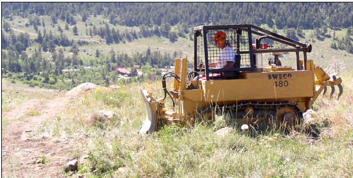
Photo 3.6 Trail maintenance prior to snowfall can help make trails smoother in the winter.
