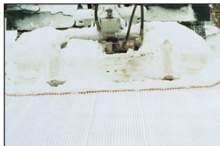
Photo 4.16 Properly finished trail
