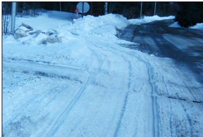
Photo 4.9 Use care to not create snow/ice buildup on railroad tracks
