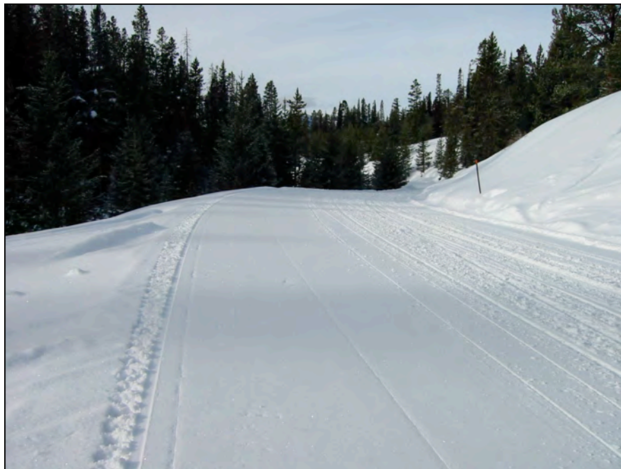
Photo 1.8 Trail grooming builds a solid, compacted base
