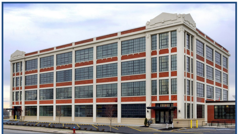
Metholatum Company Building, Buffalo, Erie Co Listed on the State & National Registers, 2017
