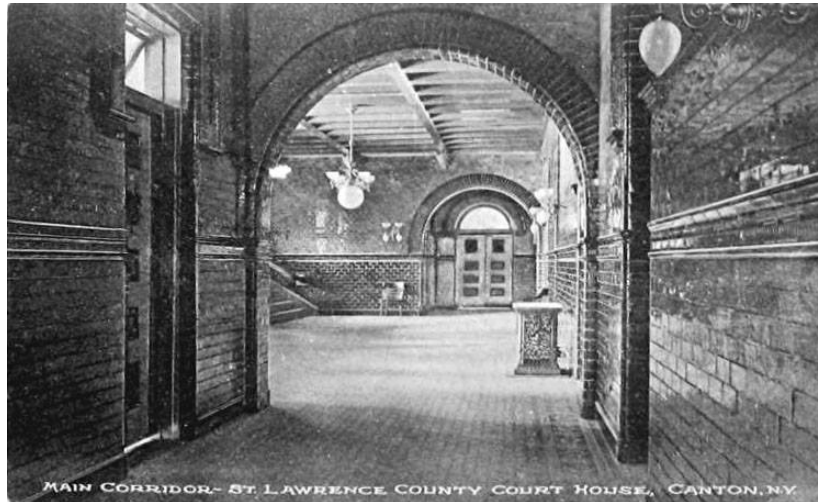
Figure 7: Photos of the re-built 1926 courthouse with fireproof tile. Via St. Lawrence County Historian.
