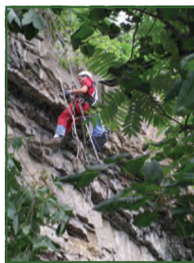
CAN rock scaler on cliff face above Whirlpool trail
