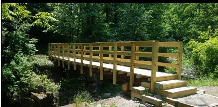
Before and after photo of the Fishkill Creek bridge at Robert H. Treman State Park. This bridge was a collaboration between the Regional Trail Crew, the Cayuga Trails Club, FORCES, and The Student Conservation Association. Photo: OPRHP
