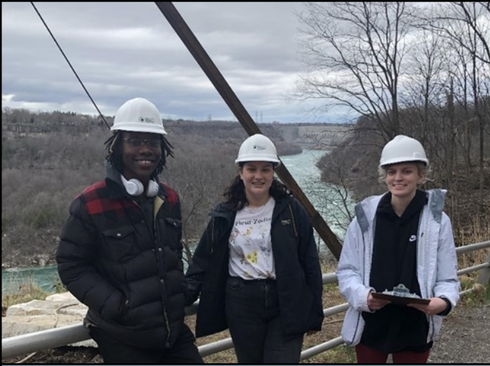
Dephil, Cassidy, and Dallas at the Whirlpool Gorge Staircase construction site. Photo: OPRHP
