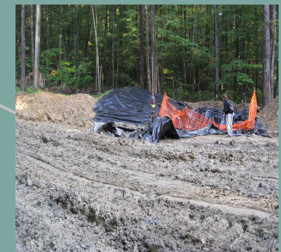
Muddy drilling road, pad site and pit.
