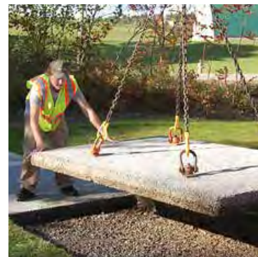
Installation of Storm-crete™ permeable unit pavers
