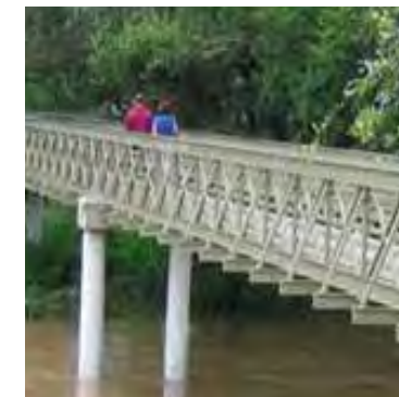
Fiberglass trail over a wetland
