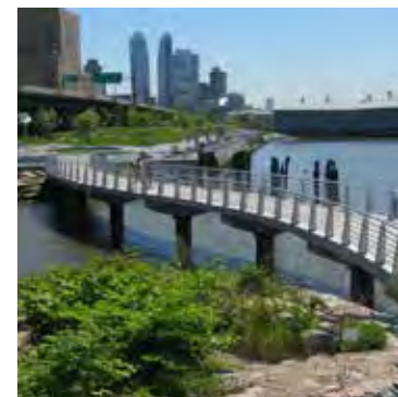
Concrete structure on piles
