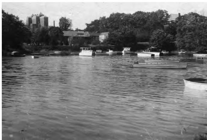
Looking back at the former hospital campus from the marina, c. 1980-1992. Image courtesy of the Kings Park Heritage Museum.
