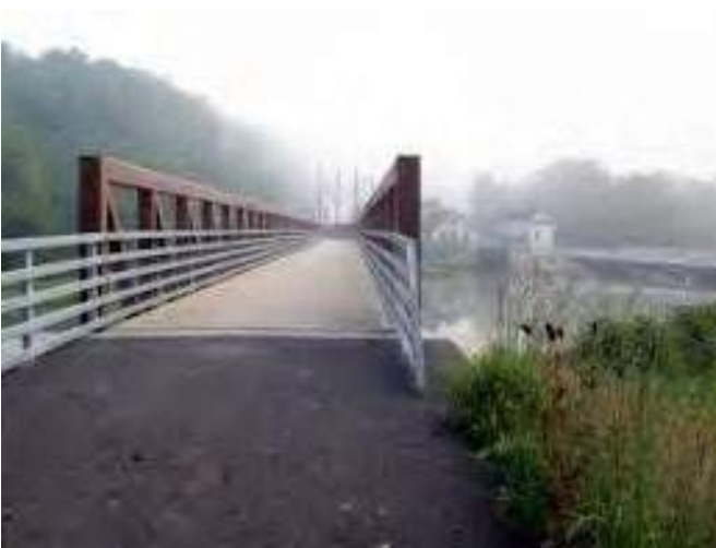
A pedestrian bridge takes trail users over the Genesee River into the Village of Mt. Morris (facing north).
