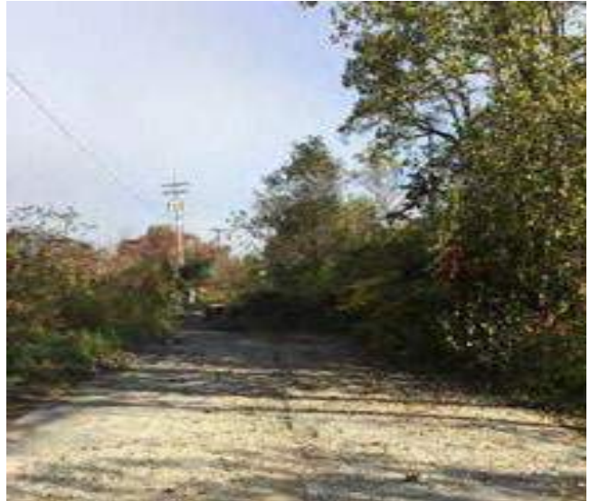
Bridge on Old Route 16, Hinsdale - facing south
