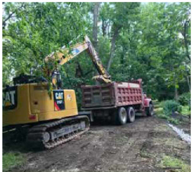
Current stonedust surfacing construction work
