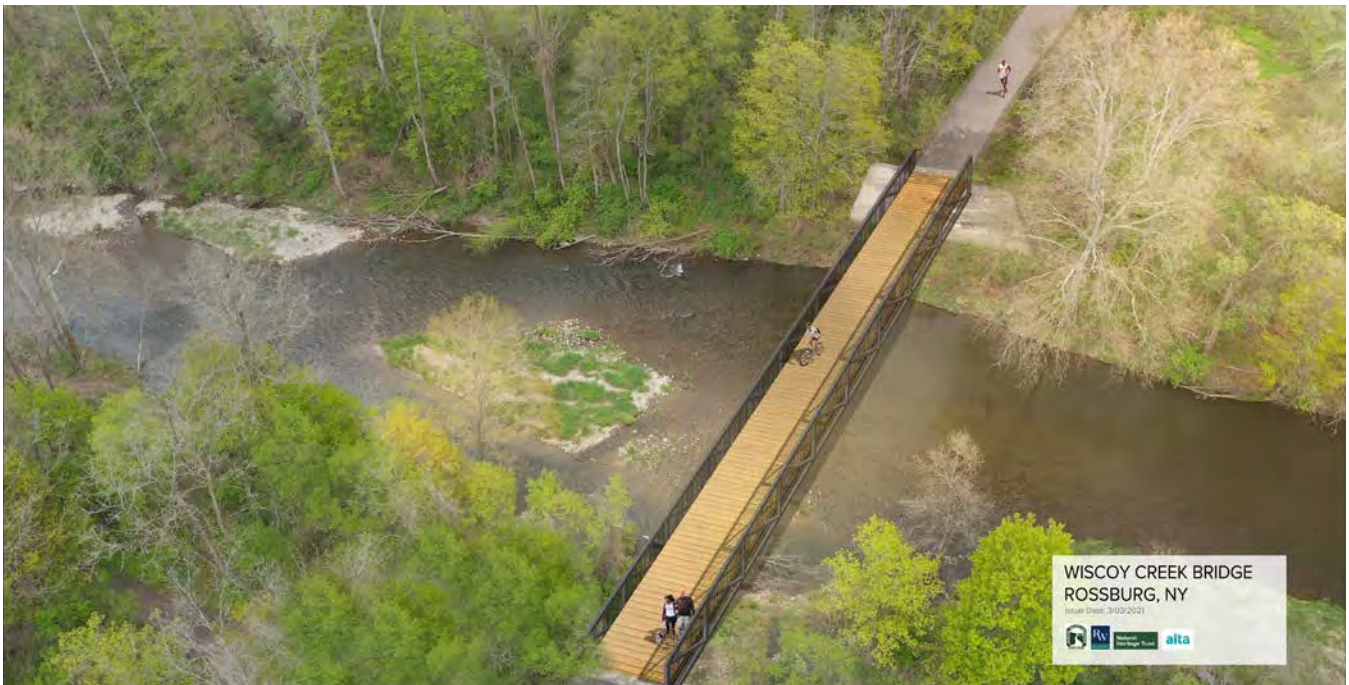
Proposed concept for a pedestrian bridge over Wiscoy Creek in Rossburg, NY
