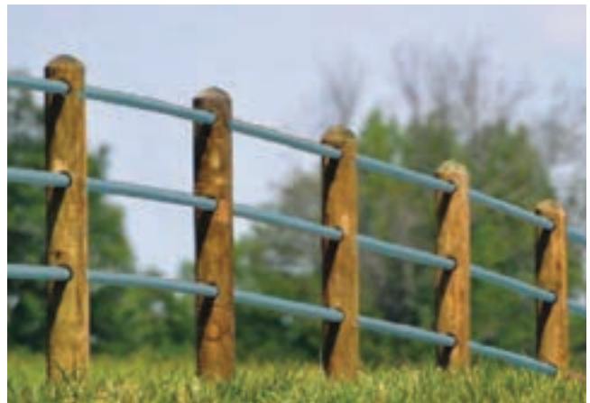
Steel rail fence
