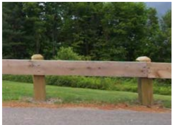
Timber guide rail fencing is a more practical application for delineating parking areas.
