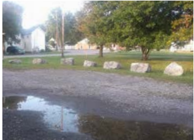
Boulder bollards being used in a parking area
