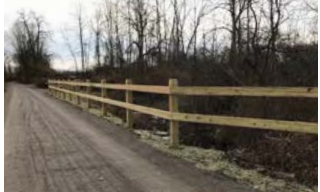
Timber fence type at Duggan Creek
