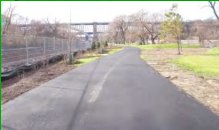
Bridge Park (under construction)
