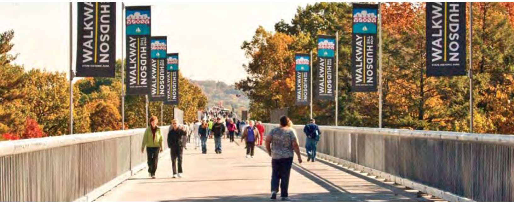
Walkway Over the Hudson State Historic Park, Poughkeepsie to Highland, NY - John Rozell, OPRHP
