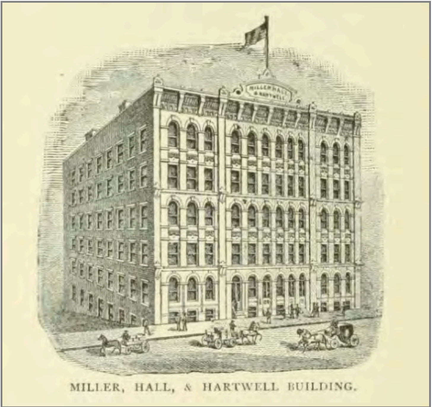
Figure 4: The collar factory ca. 1886 prior to the construction of the addition in 1891 (source: Arthur James Weise, The City of Troy and Its Vicinity [Troy: E. Green, 1886] 274).
