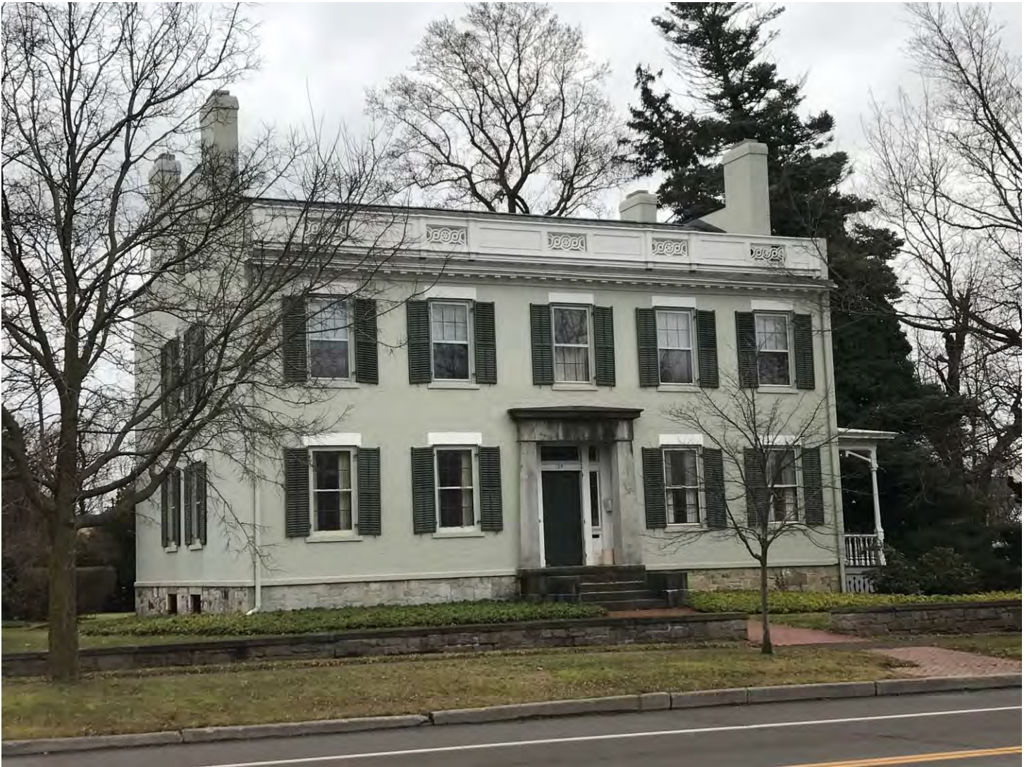
Figure 8. 29 Gibson Street, Canandaigua. Site visit photograph 2024 by Saralinda Hooker, Preservation Consultant.
