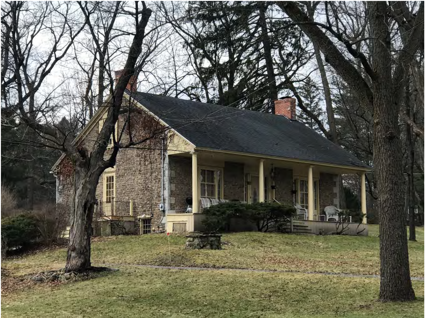
Figure 6. Cobblestone residence at 5037 Butler Road, Canandaigua. Site/Survey photograph by Saralinda Hooker, Preservation Consultant.
