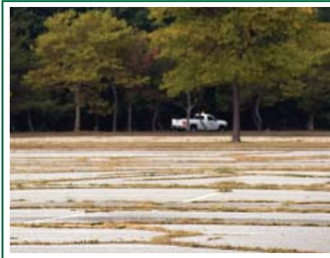
Parking lot at Clarence Fahnestock State Park
