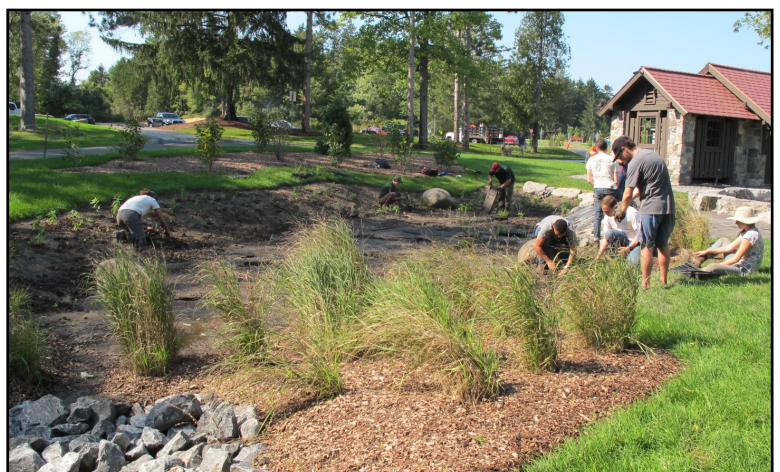
SUNY ESF FORCES working in a bioswale at Green Lakes State Park planting sprouts established by the Plant Materials Program.
