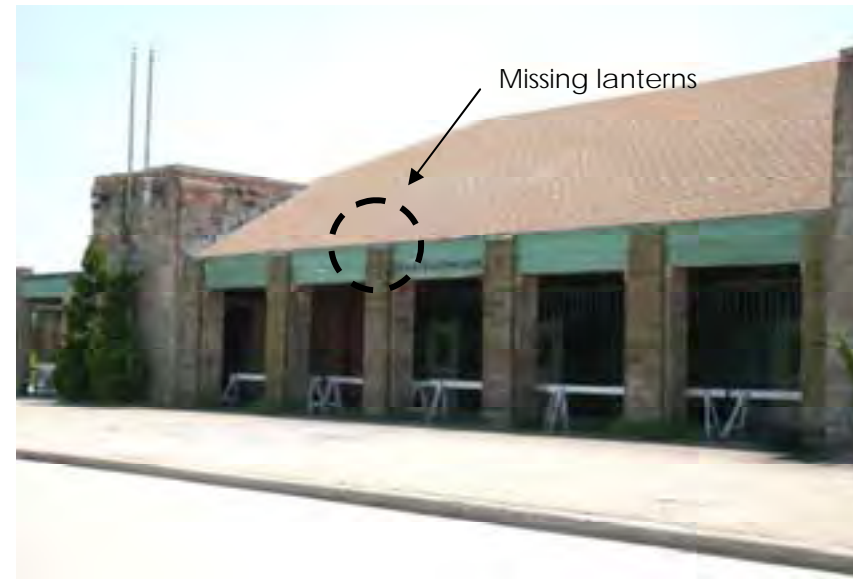
North building façade (2013)
