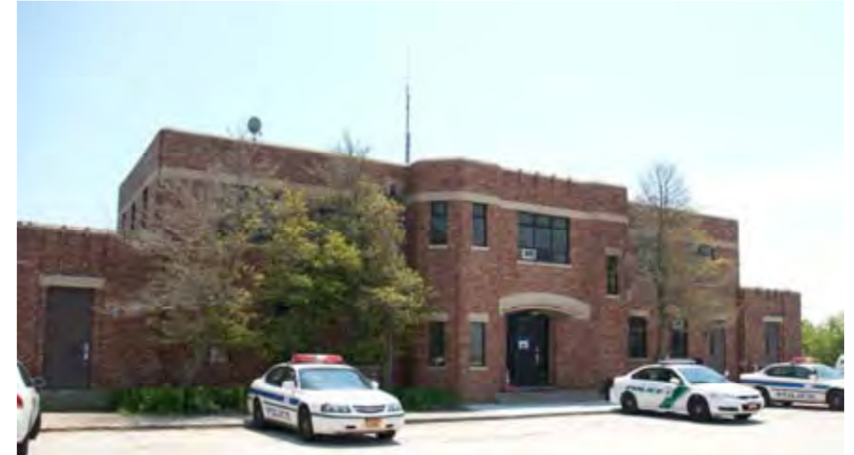
Police Headquarters' - north elevation 2013
