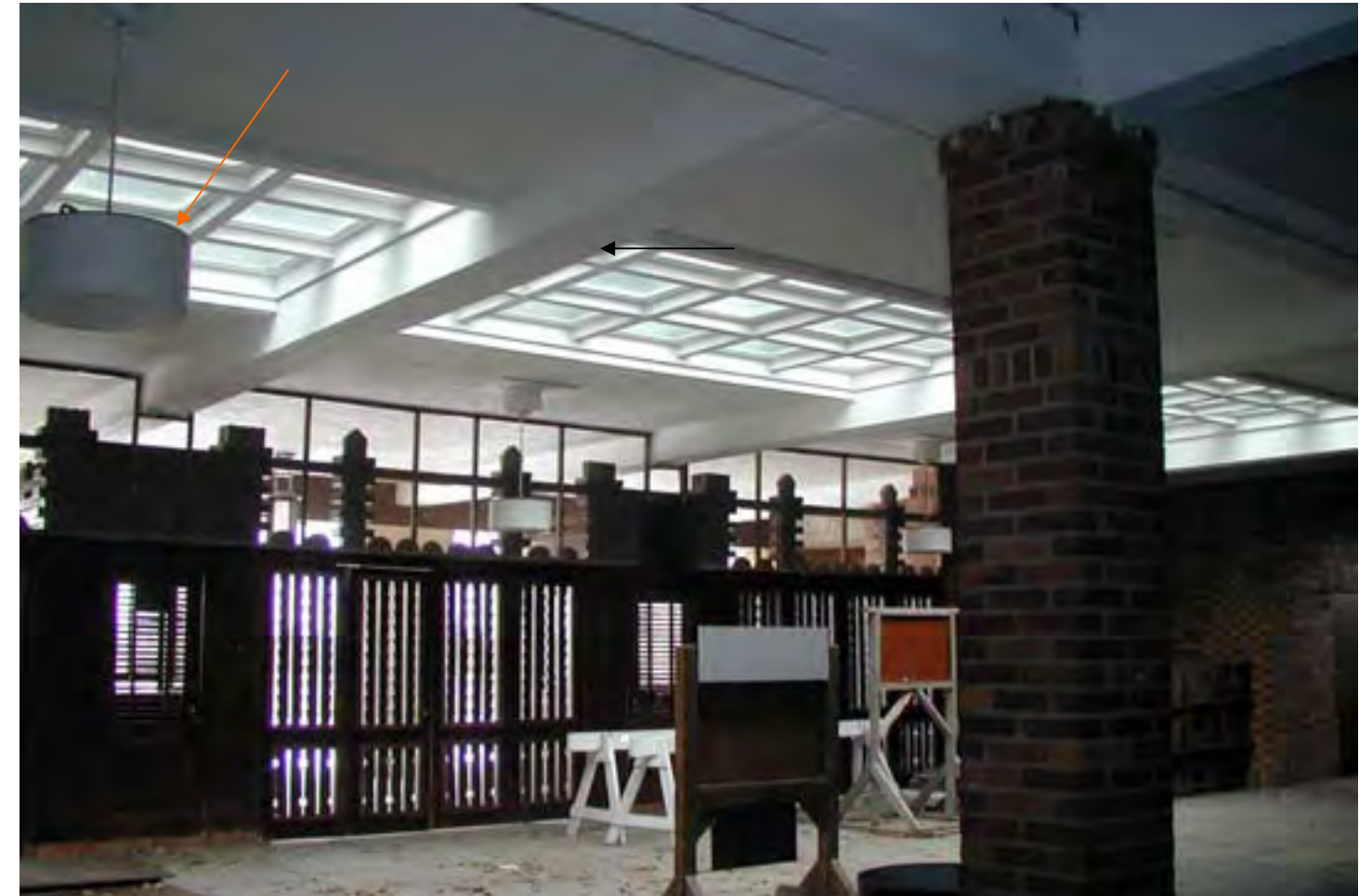
North Lobby—2009. Note painted ceiling and woodwork and replacement lighting.
