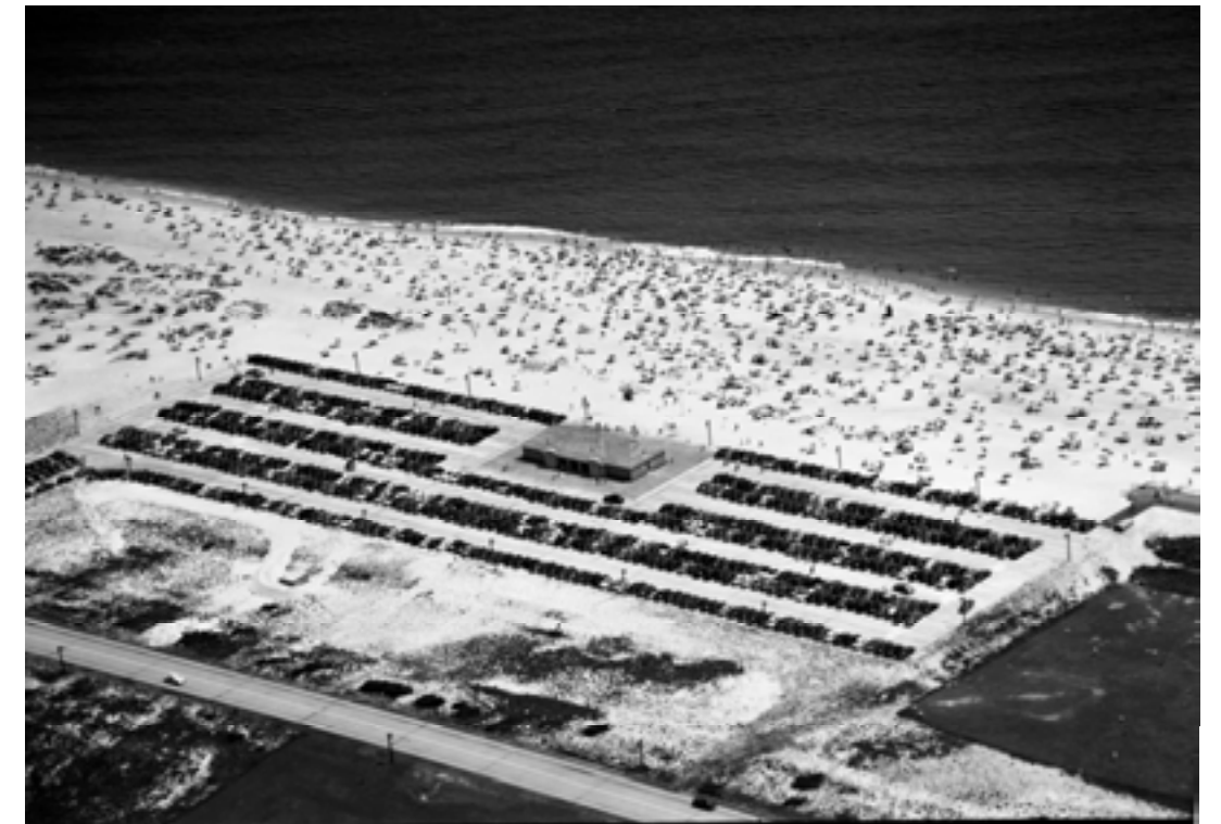
Parking Field & Comfort Station 2, 1960's
