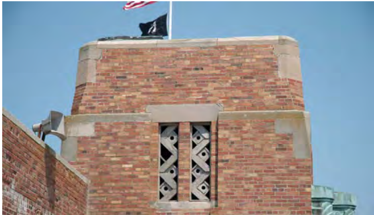
West Mall Building Tower 2013. Note Barbizon Brick, sandstone and Art Deco details.
