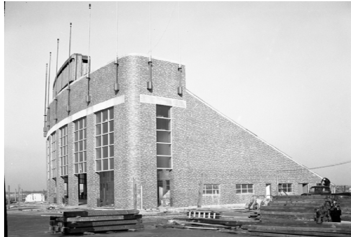
Marine Theater, Amphitheater under construction, c. 1949-52.
