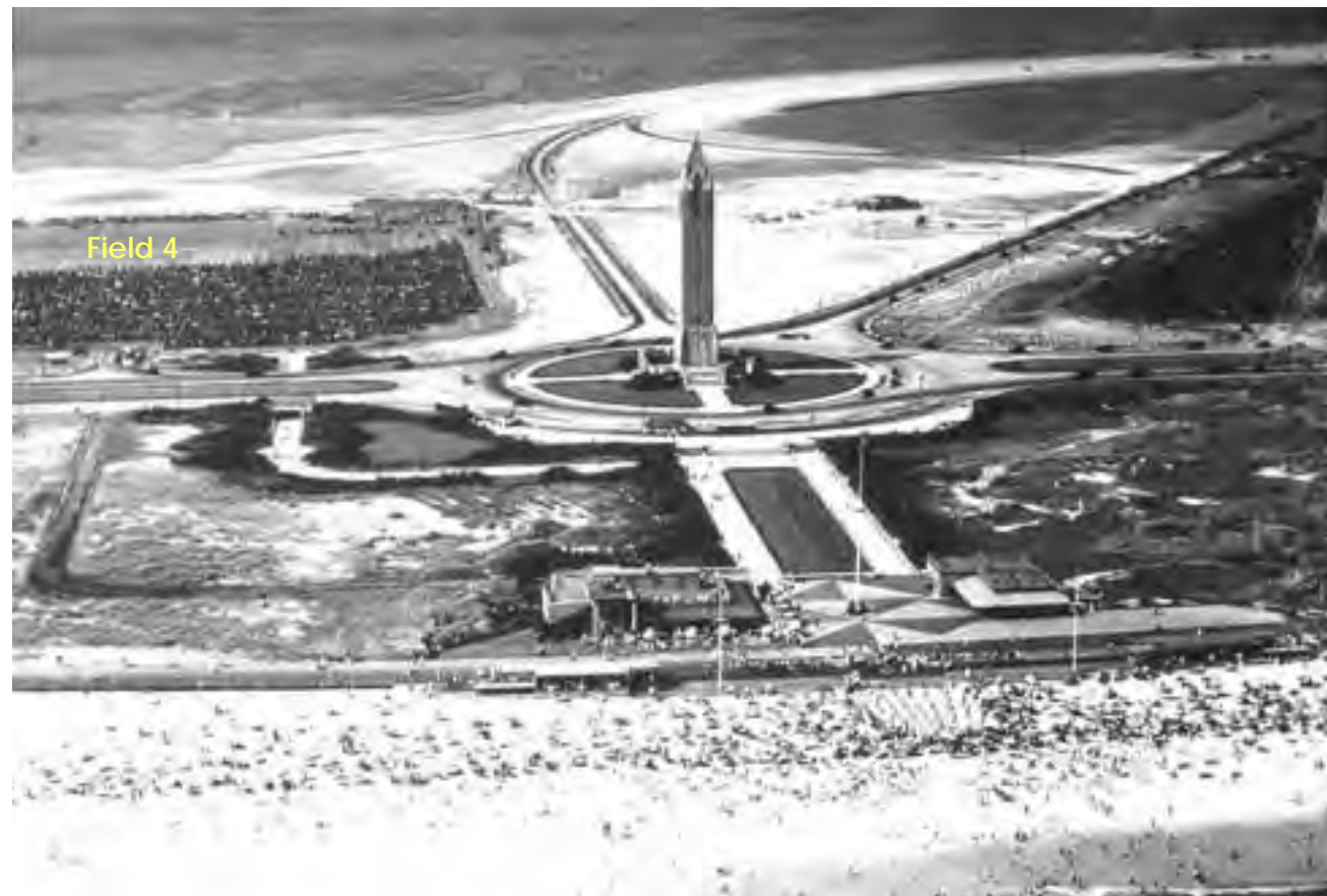
Aerial View c. 1932. Field 4 complete, Field 5 under construction
