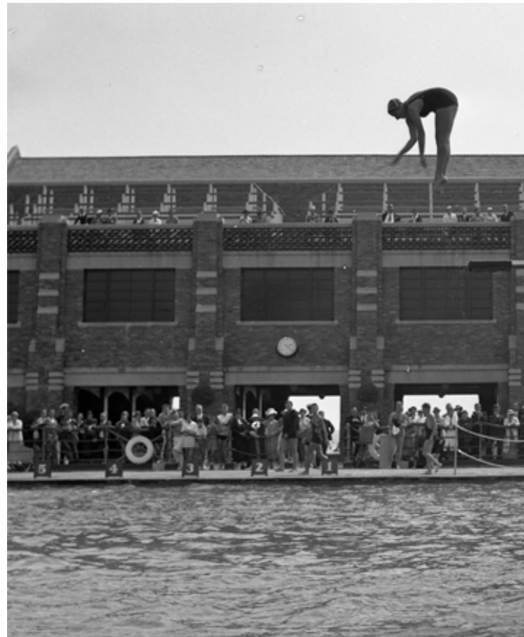
Detail of North Elevation (1930's). Note the open passages in the central bays of the building. The concession counters lined the outside walls of the large open interior space. The open passages allowed a clear view of the ocean from the pool courtyard.
