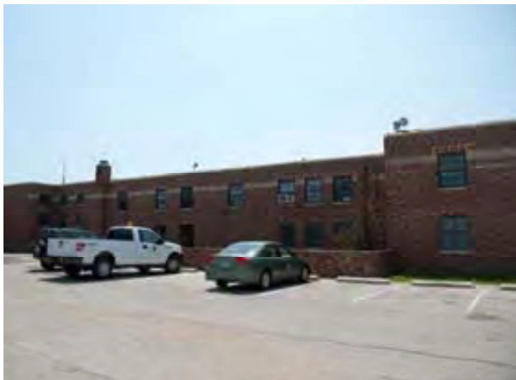
Administration Building, East Façade 2013
