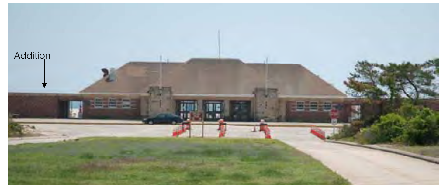
Comfort Station, north elevation 2013
