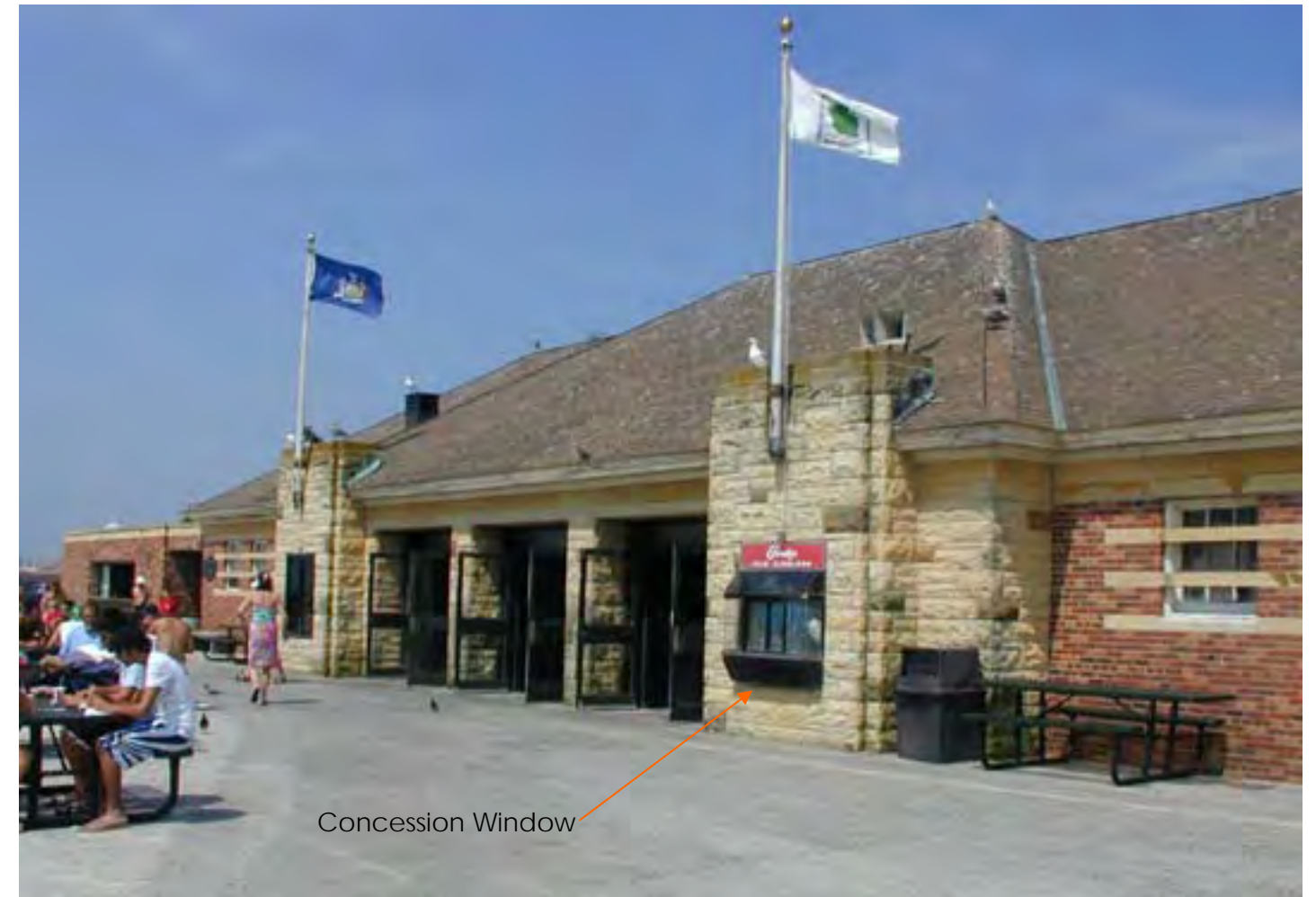
Comfort Station, south elevation 2009
