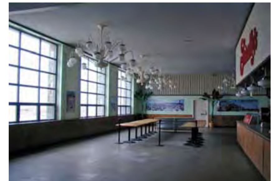
West Bathhouse, Terrace level concession 2009
