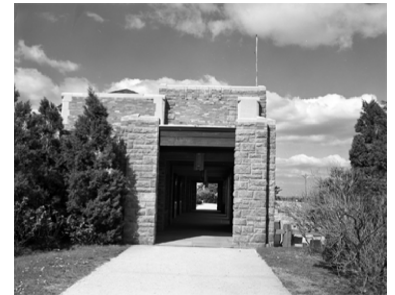
North Building, East Elevation of Loggia c.1970
