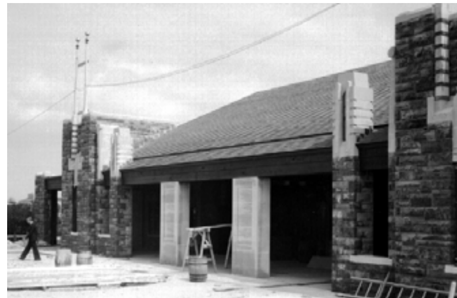
North Building, North Elevation under construction c.1930.
