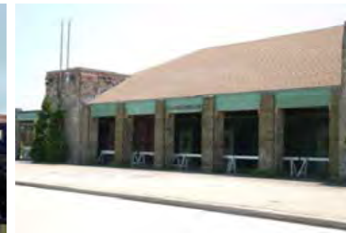
East Bathhouse, North Elevation 2013
