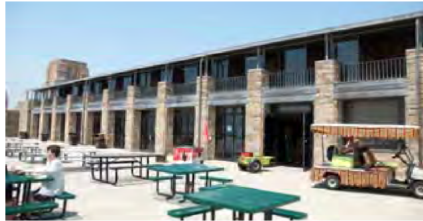
East Bathhouse, South Elevation 2013. Note: removal of awnings & partial enclosure of sundeck.
