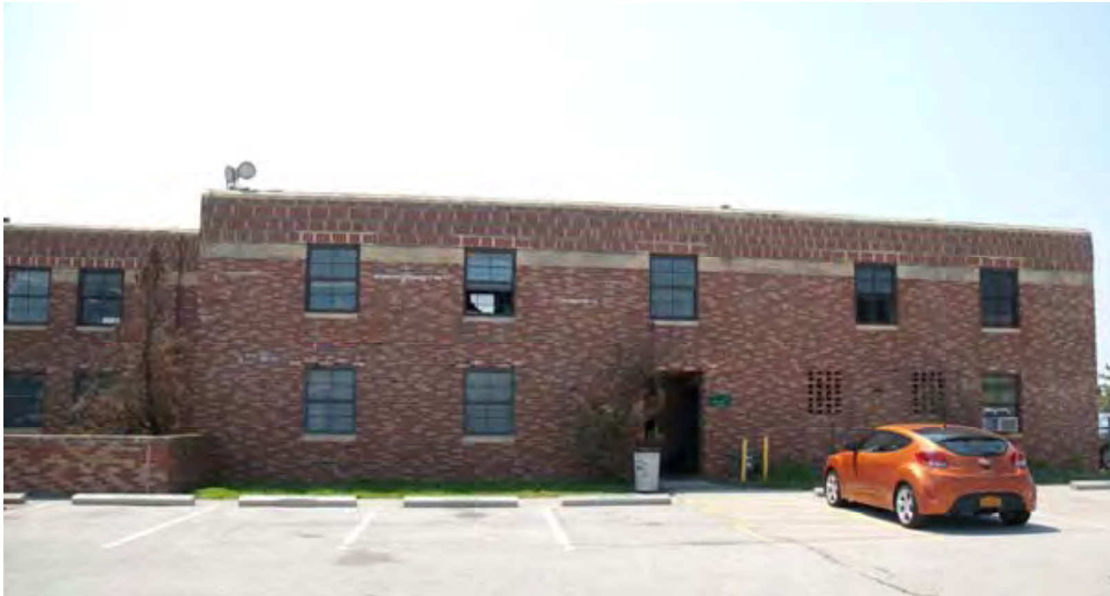
Administration Building, East Façade 2013
