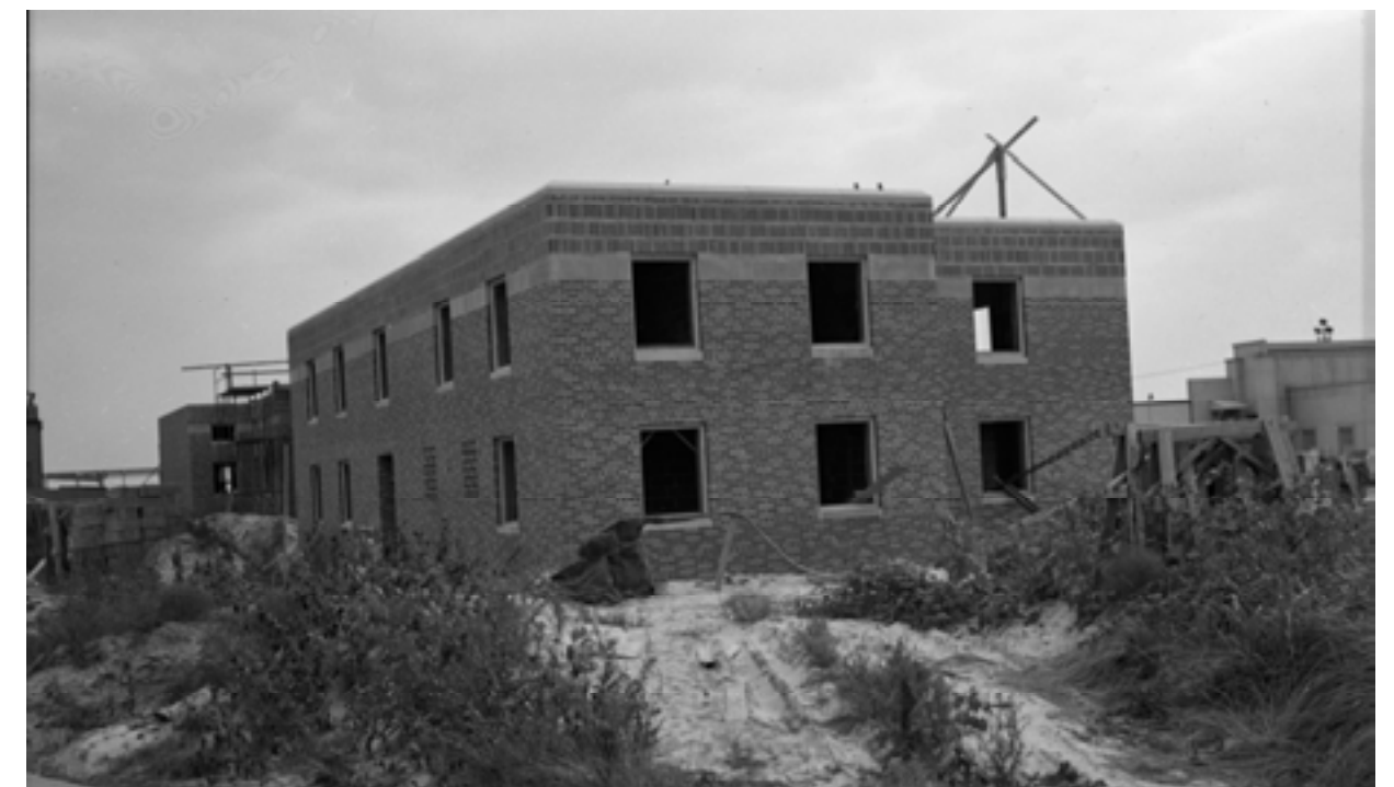
Administration Building under construction c. 1950-1951.
