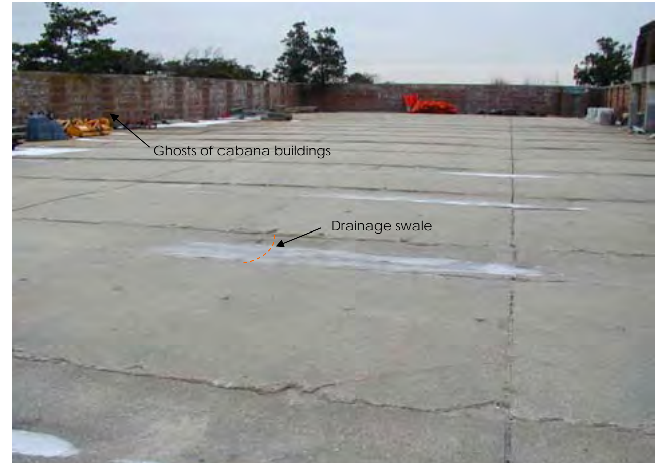
Outer Courtyard—Former changing area c.2009.
