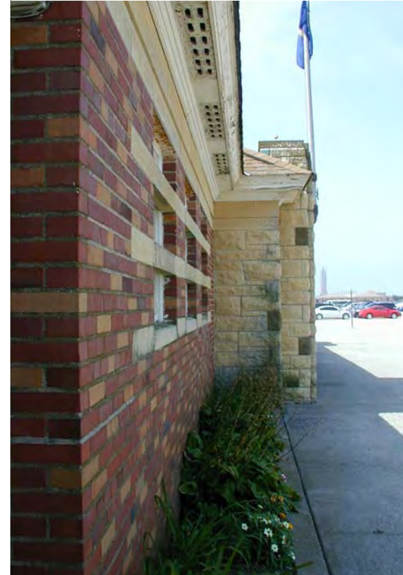
Sandstone Tower & Planting Bed, 2013
