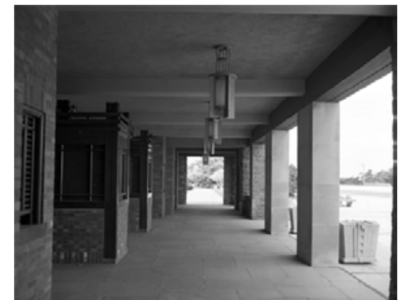
North Building, Loggia c.1970. Note Art Deco Chandeliers
