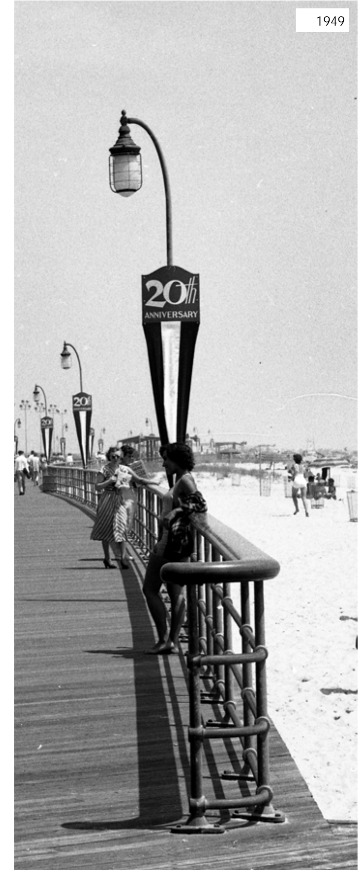
Boardwalk Railing—note wood hand rail.
