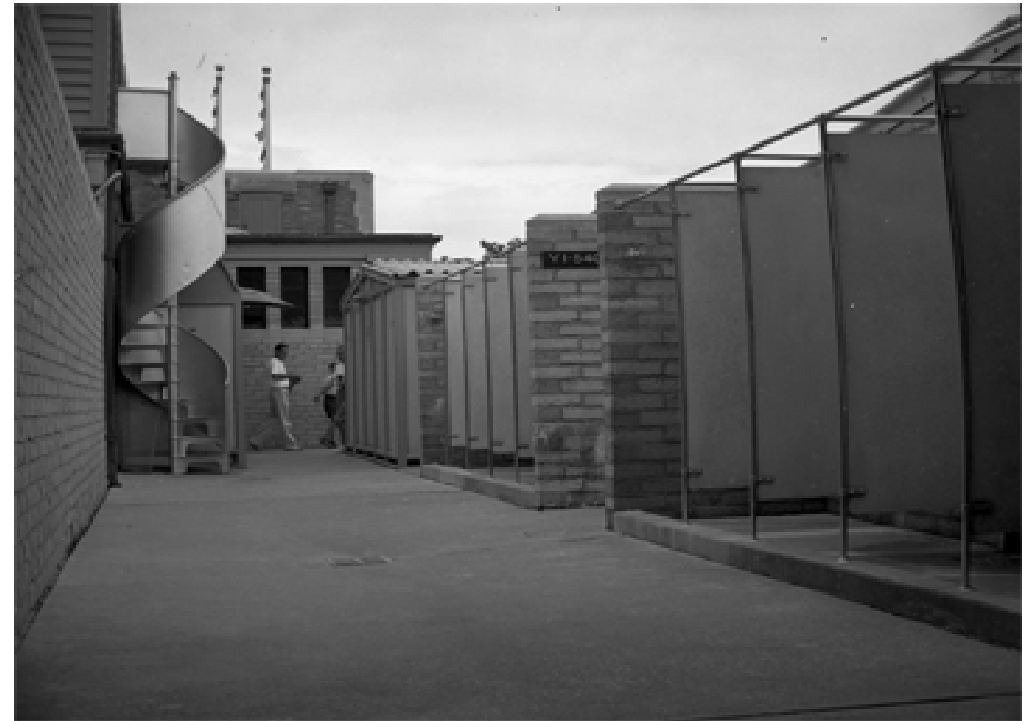
Changing Rooms with spiral staircase (1930's)
