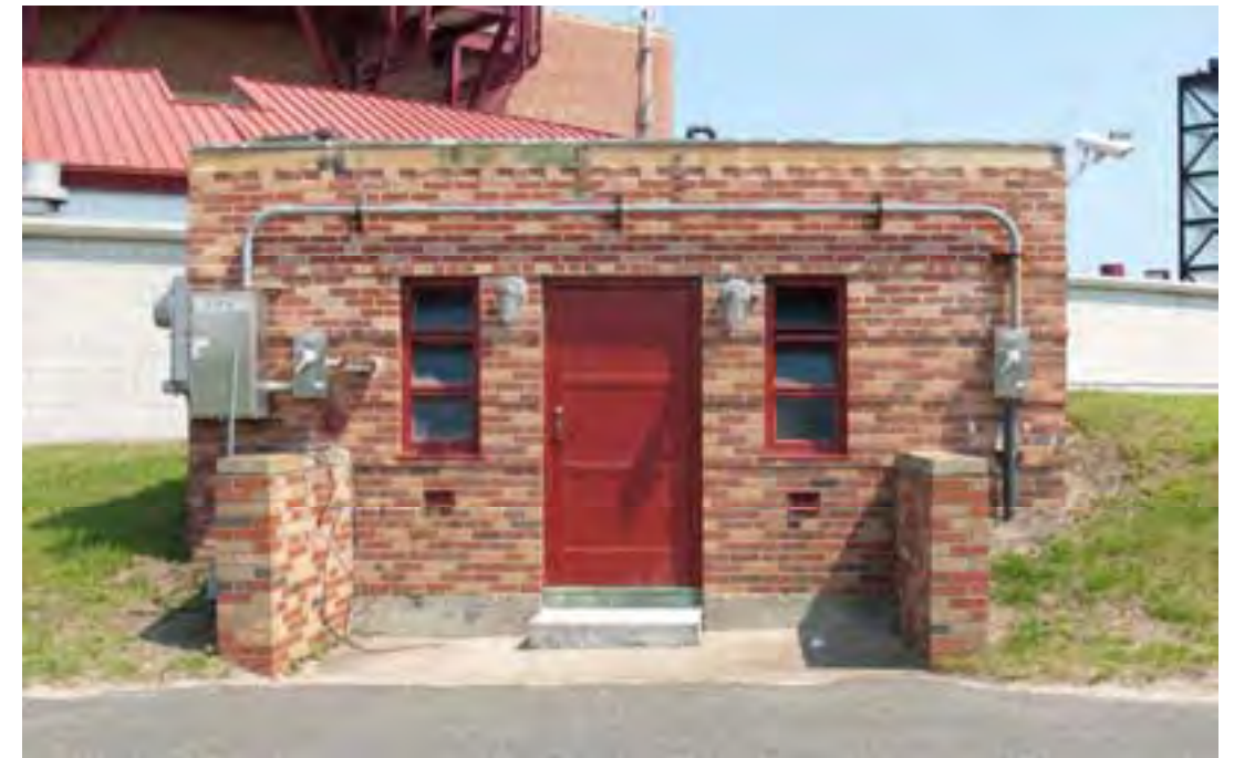
Transformer Vault, Marine Theater, 2013
