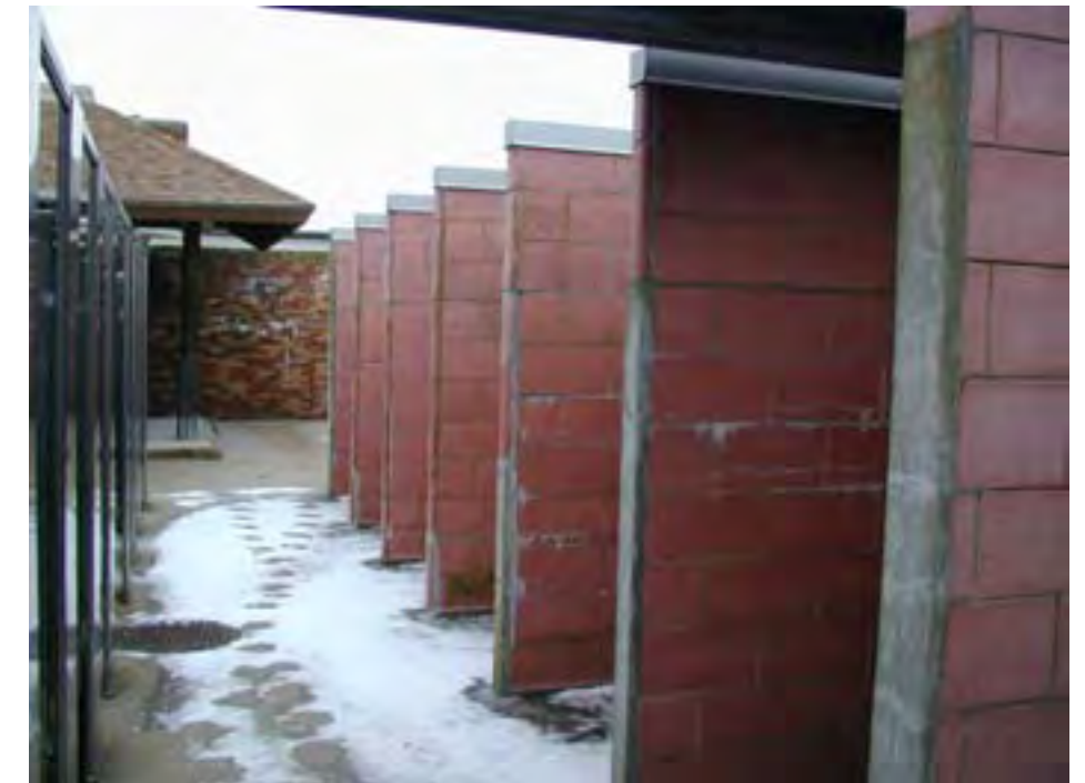
Outer Courtyard—1980's Showers c.2009.
