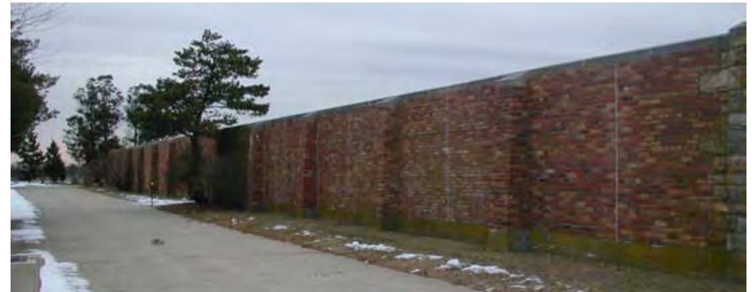
Brick screen wall 2009
