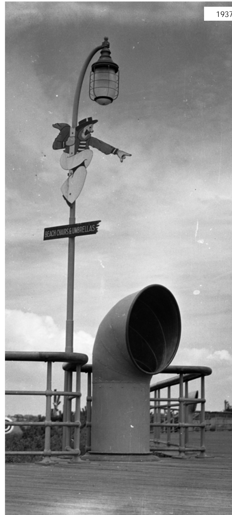
Boardwalk Fire Suppression System & Light Pole with signage
