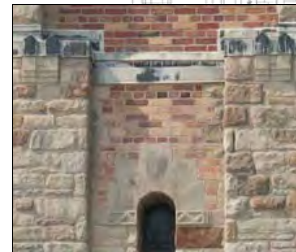
East Bathhouse, Detail of south tower (2013)
