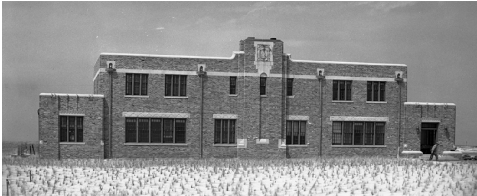
Police Headquarters' under construction (south elevation) 1937.
