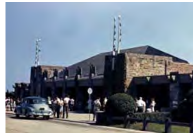
East Bathhouse, North Elevation 1940's
