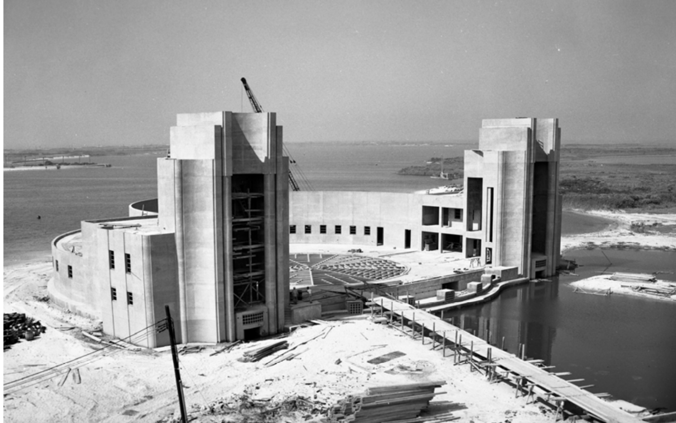
Marine Theater, Amphitheater stage under construction, c. 1949-52.
