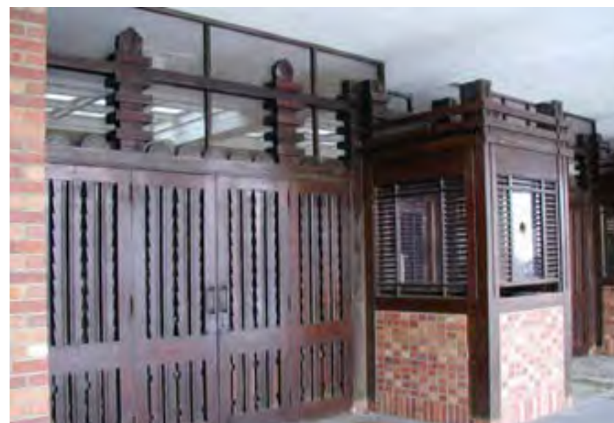
North Building, Loggia—Wood Screen Wall 2009.
