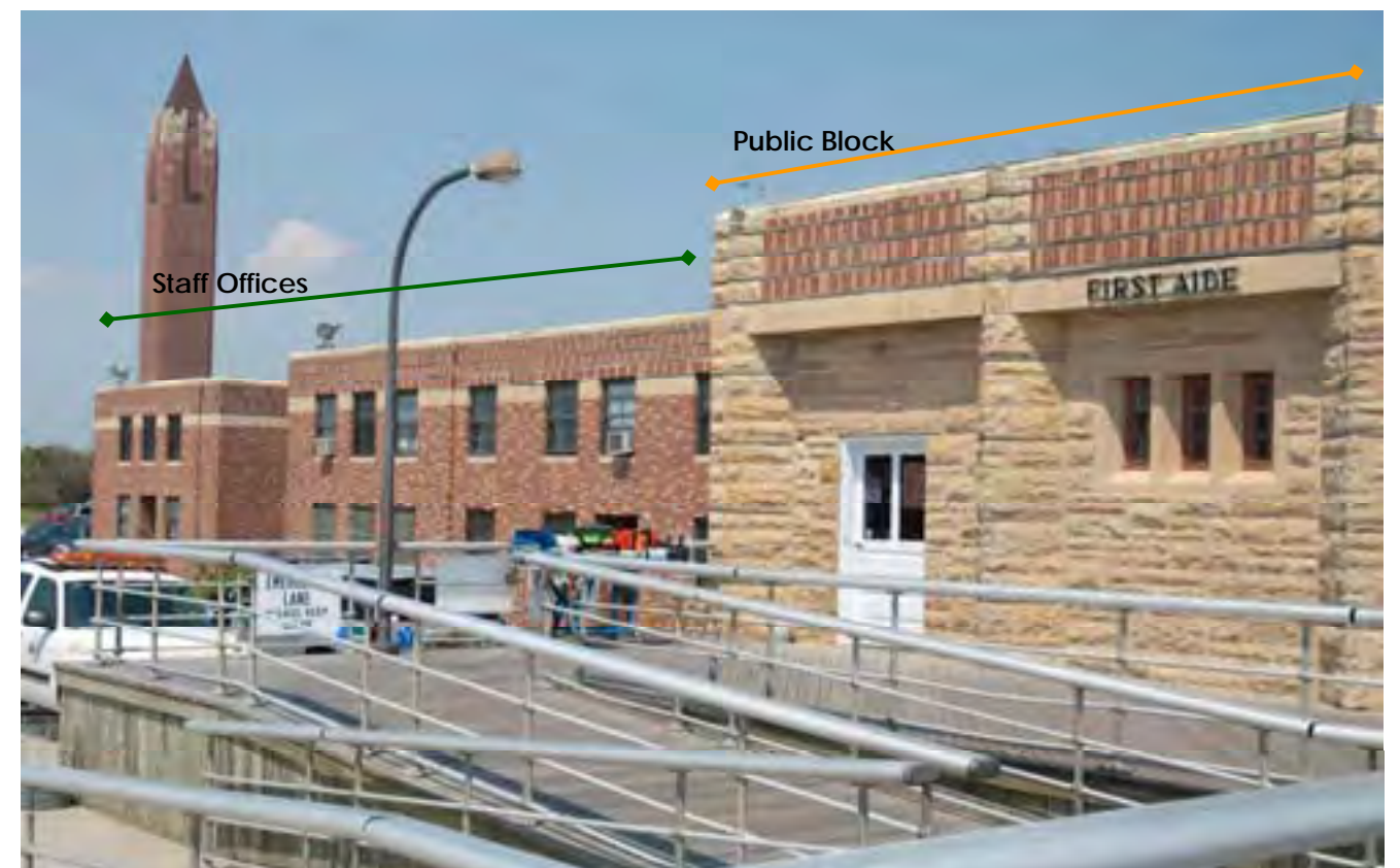
Administration Building—West Façade (2013). Note the transition between the public 'block' of the building (front -right) and the Park's staff section of the building (rear). The First Aide Station on the Boardwalk is primarily constructed on coursed sandstone with decorative trim and projecting piers. The block to rear is much more simply executed with Barbizon brick with limited sandstone trim.
