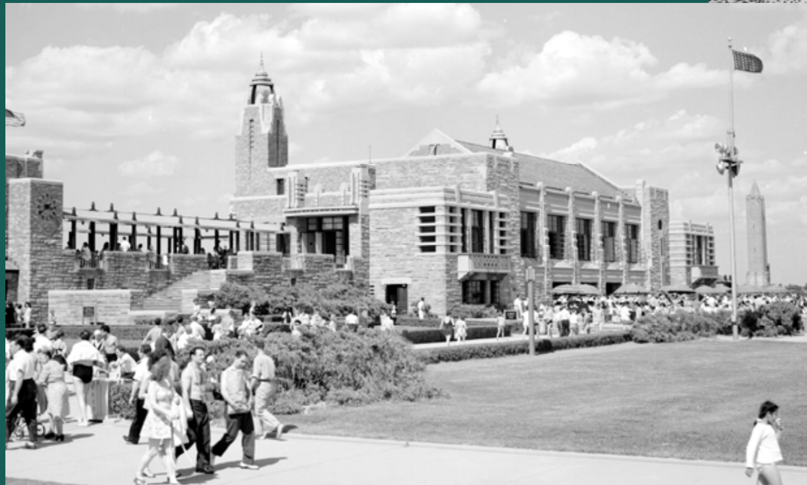
South Elevation: West Bathhouse 1950's
