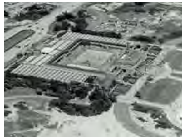
Aerial View of West Bathhouse (1930's)
