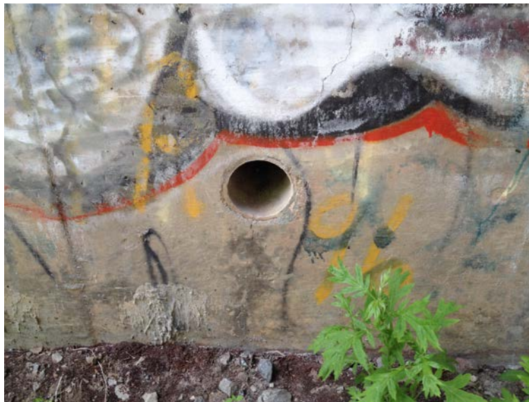
Photo 4: BIN 1068229. View of the cementitious drain pipe.
