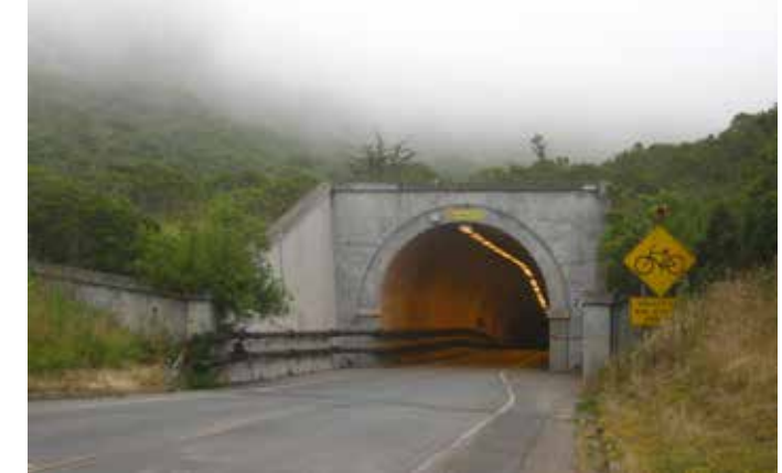
Cyclist-activated warning signage with flashing beacon to notify drivers about presence of cyclists in tunnel
