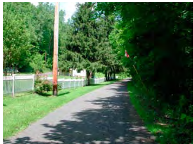
Fencing matching an adjacent landowner's fence installed along the Finger Lakes Region's Catharine Valley Trail, in Schuyler and Chemung Counties, to separate trail and private property.
