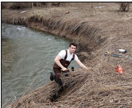
Charlie Ippolito planting native trees and shrubs to stabilize the stream bank at Ganondagan State Historic Site. Photo: OPRHP
