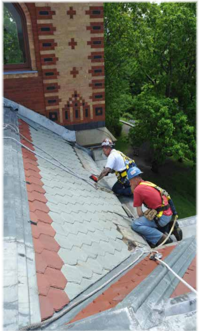
Repairing the roof at Olana State Historic Site
