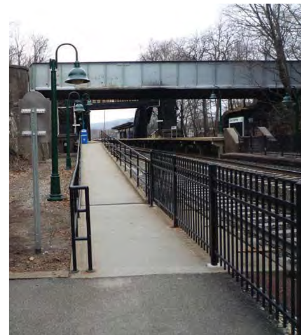
Northbound platform path facing south
